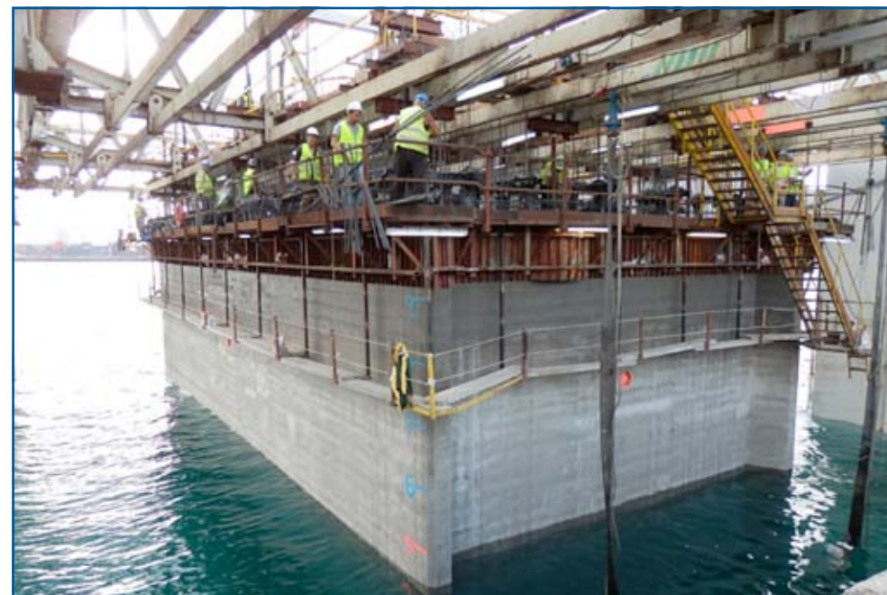
Mar del Teide floating dyke
