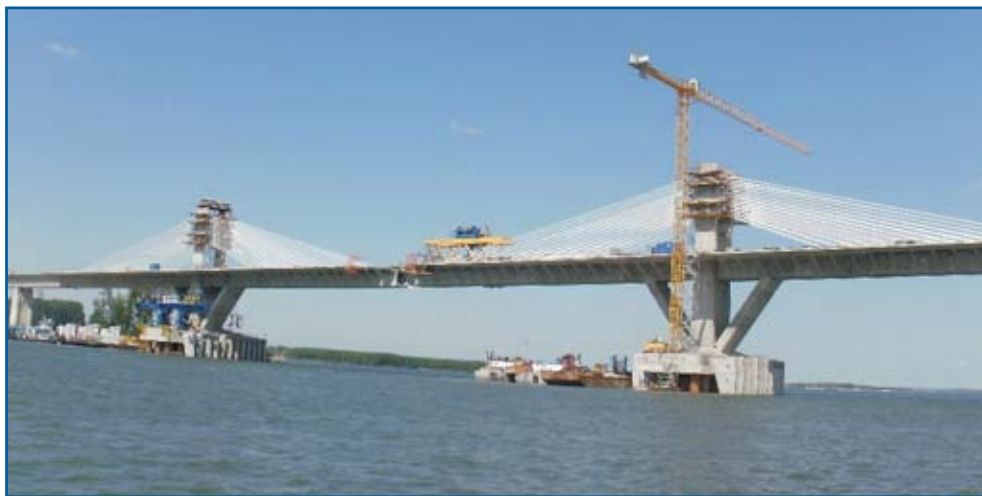
Vidin-Calafat Bridge (Bulgaria-Romania)
