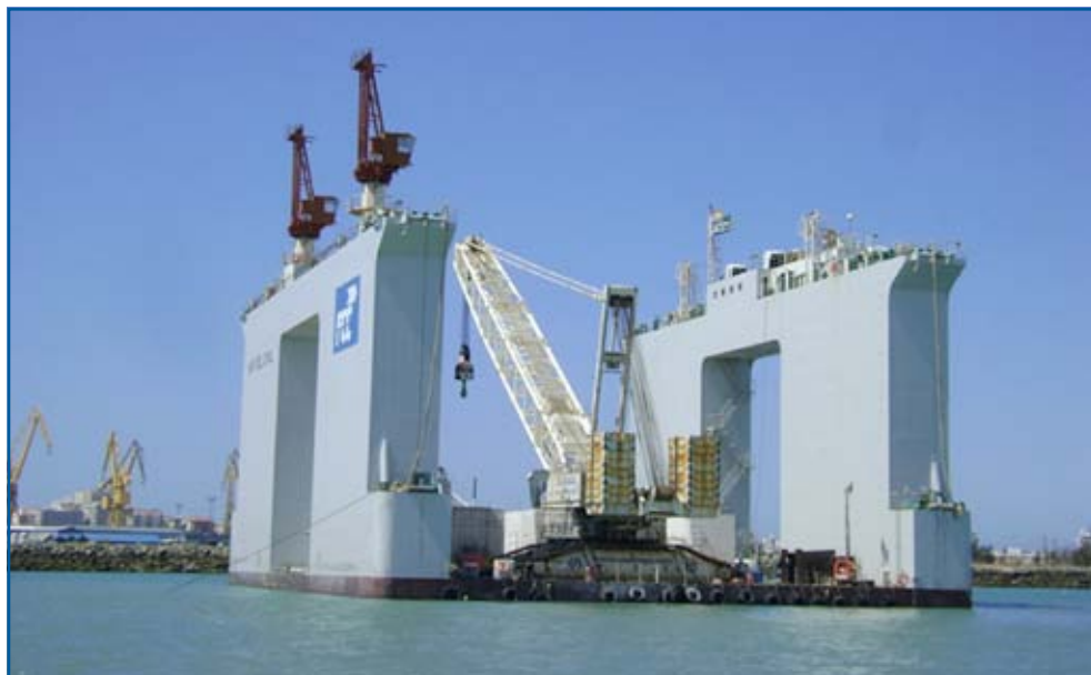
Mar de Enol floating dyke. New Container Terminal in Cádiz
