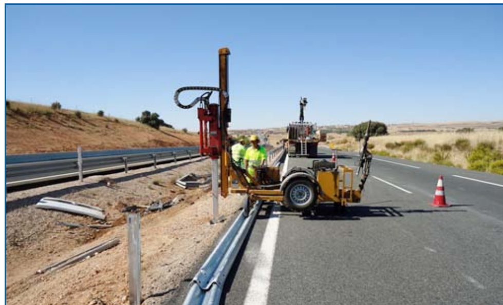
Installing safety fences on highways
