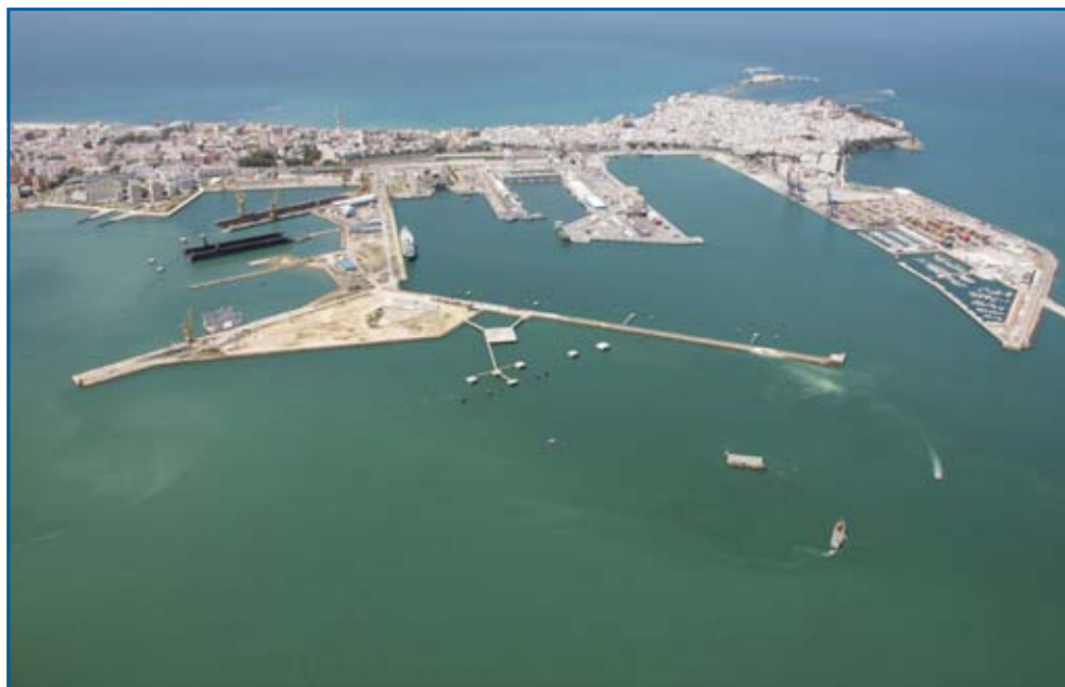
Cadiz Port Container Terminal
