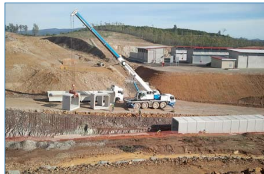
Placement of modular reinforced concrete structures
