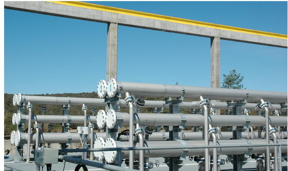
Ultrafiltration membrane bioreactor (MBR).
