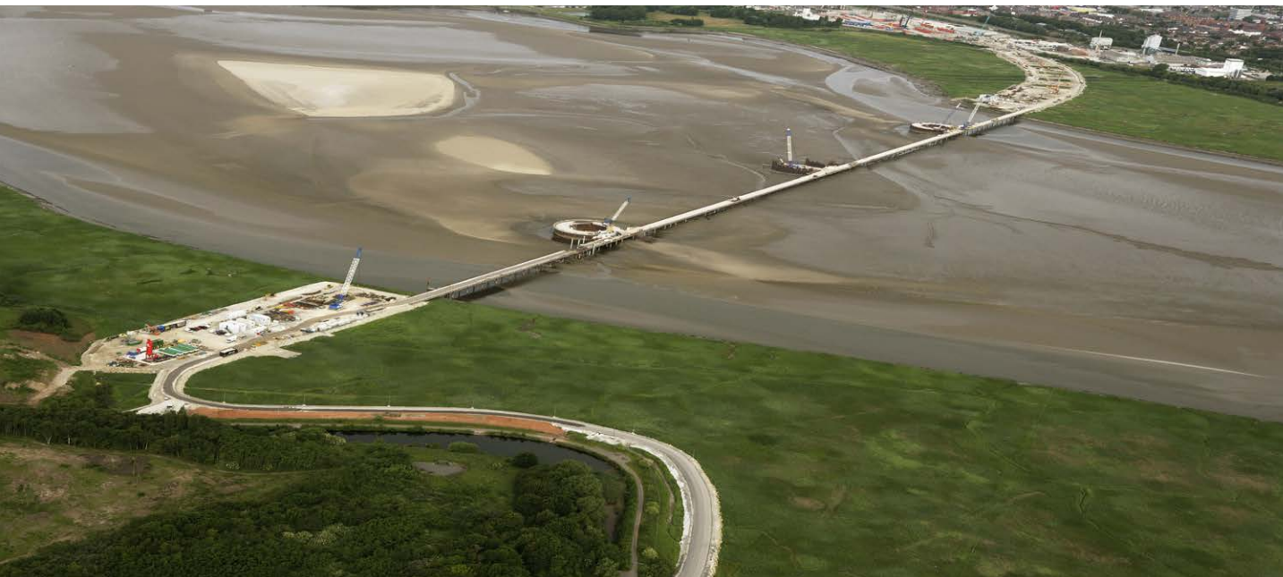
Mersey Viaduct (UK).
