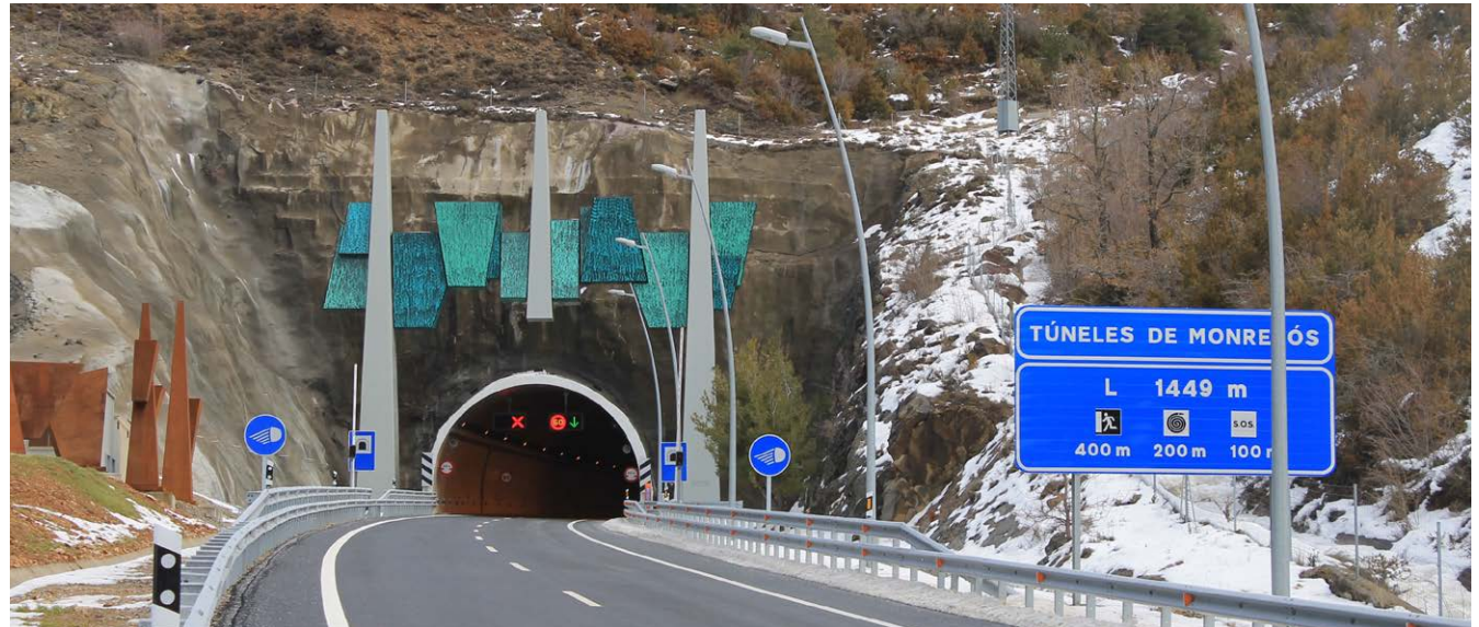
Integration of Road Tunnel Control Systems. Monrepós, Huesca (Spain).
