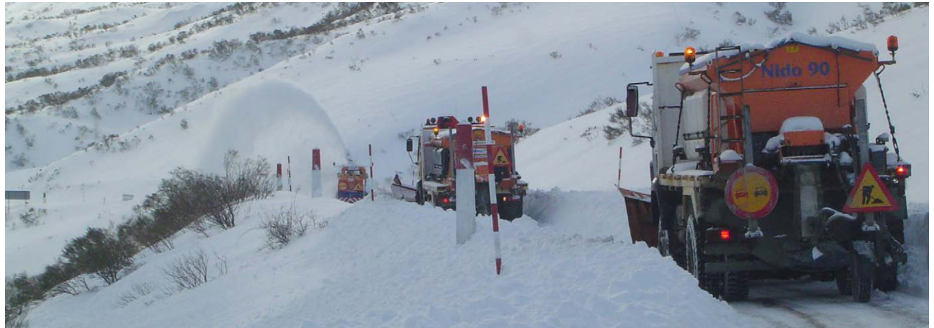
Conservation and maintenance work.
