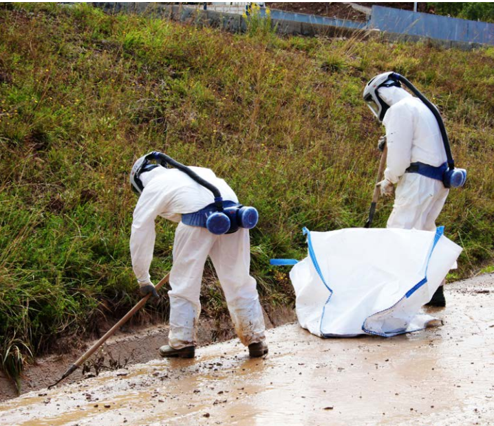
Soil decontamination activity in Bailín, Huesca (Spain).
