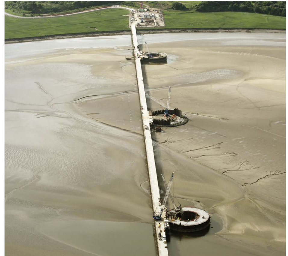
Mersey Bridge (UK).
