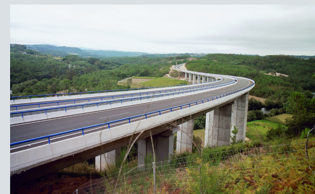
Viaduct over the Ulla River, Galician Motorway
