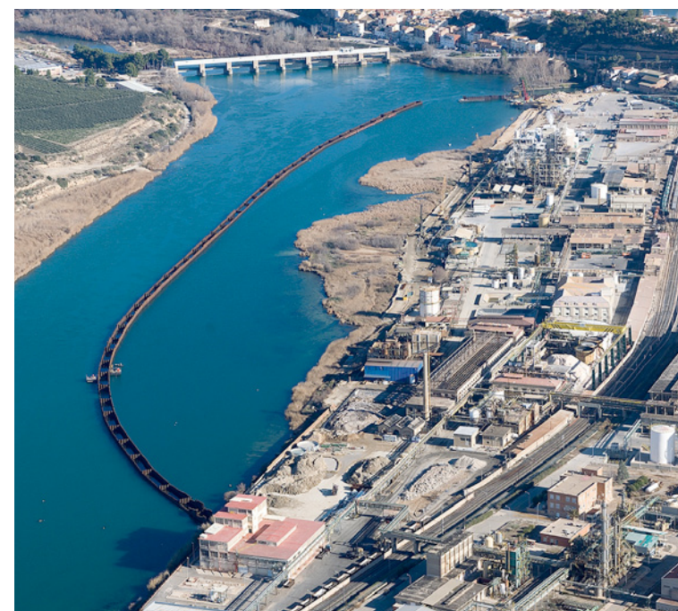
Decontamination of Flix Reservoir, Tarragona
