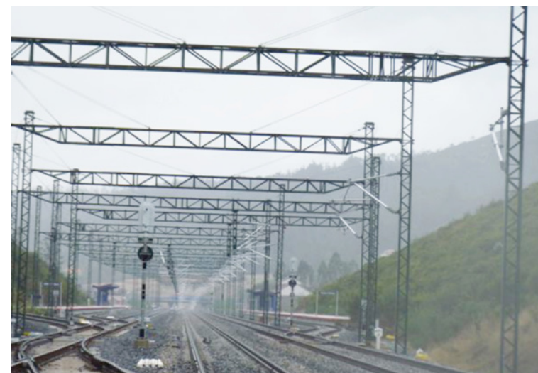
Catenary on the high-speed Atlantic Artery
