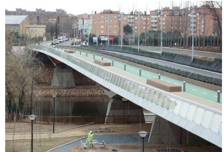
Bridge over the Pisuergra River, Valladolid
