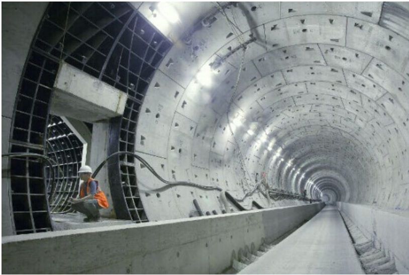
London Crossrail Tunnel (Photo credit: LCR)
