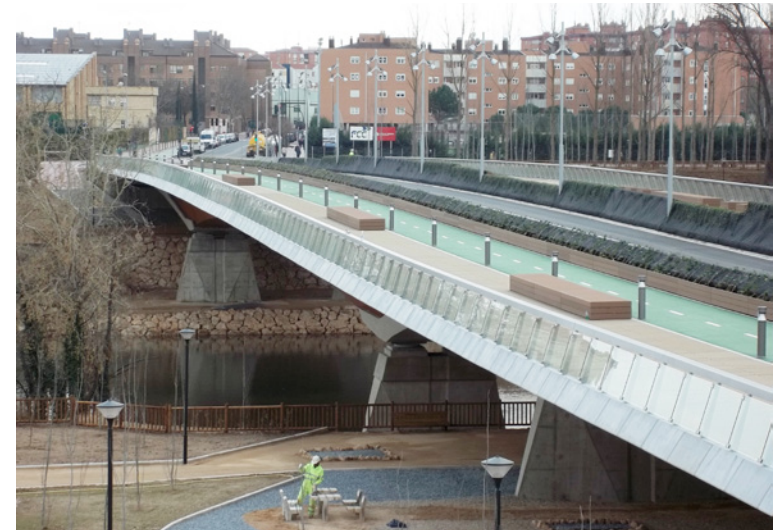
Bridge over the Pisuergra River, Valladolid
