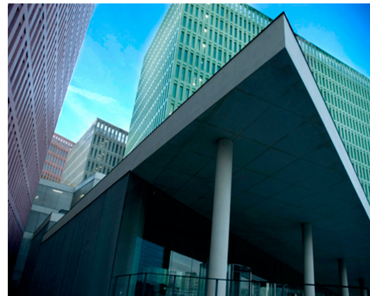
City of Justice complex in Barcelona
