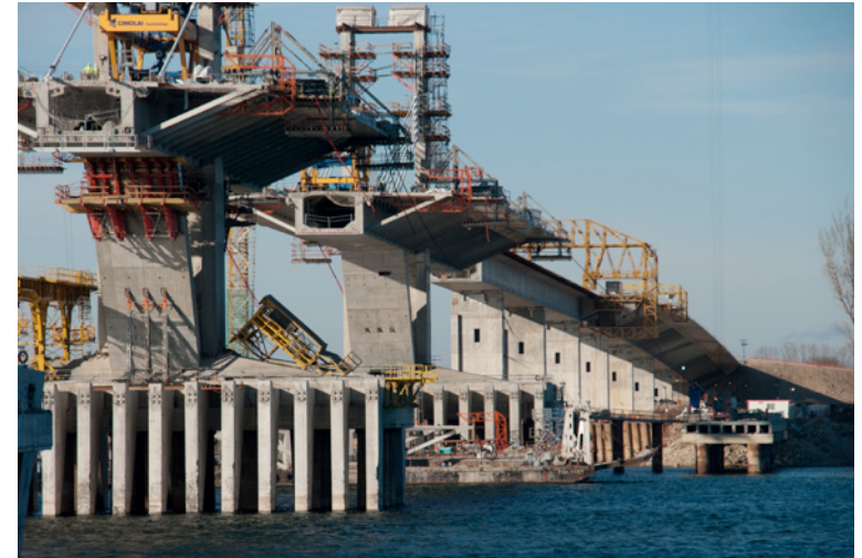
Vidin-Calafat Bridge between Romania and Bulgaria
