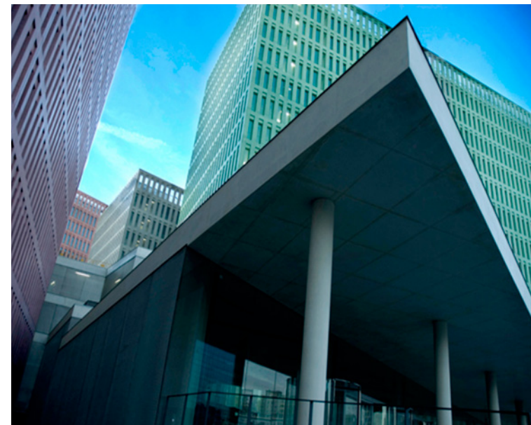
City of Justice complex in Barcelona
