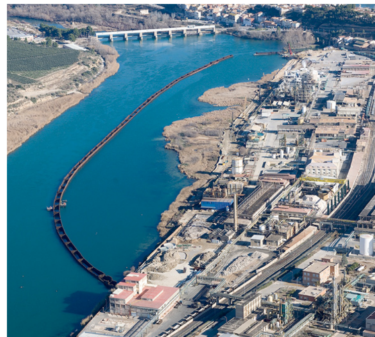
Decontamination of Flix Reservoir, Tarragona
