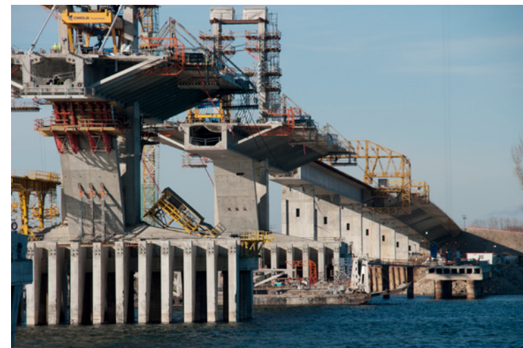
Vidin-Calafat Bridge between Romania and Bulgaria
