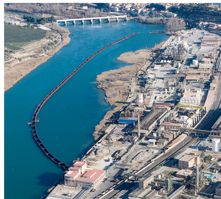
Decontamination of Flix Reservoir, Tarragona
