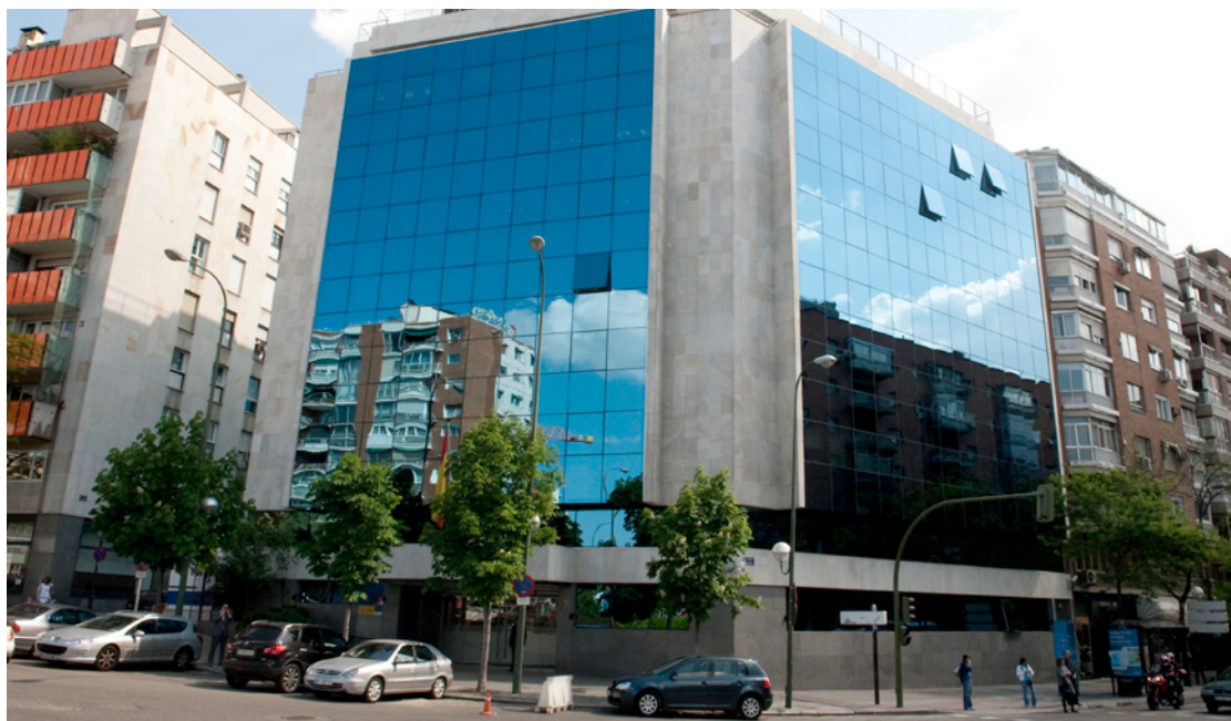
Road Infrastructure's General Direction headquarters rehabilitation, Madrid
