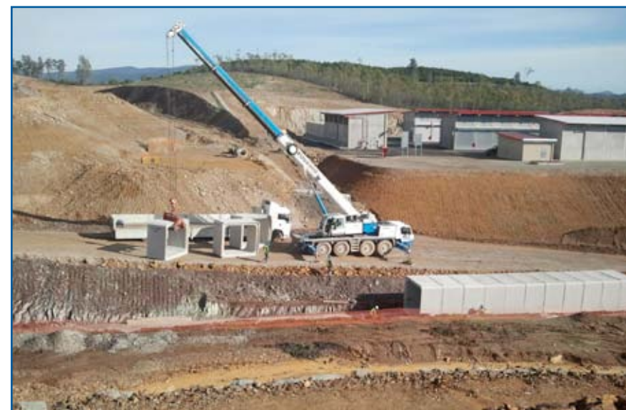
Placement of modular reinforced concrete structures
