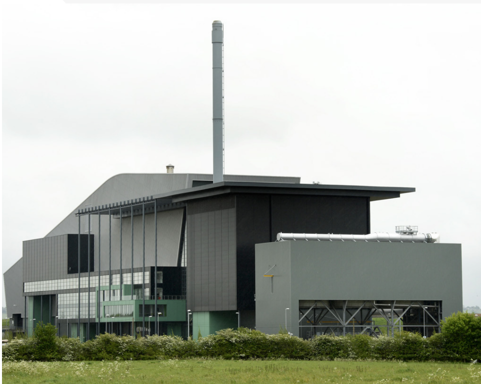
Incineration plant in Lincolnshire (United Kingdom).
