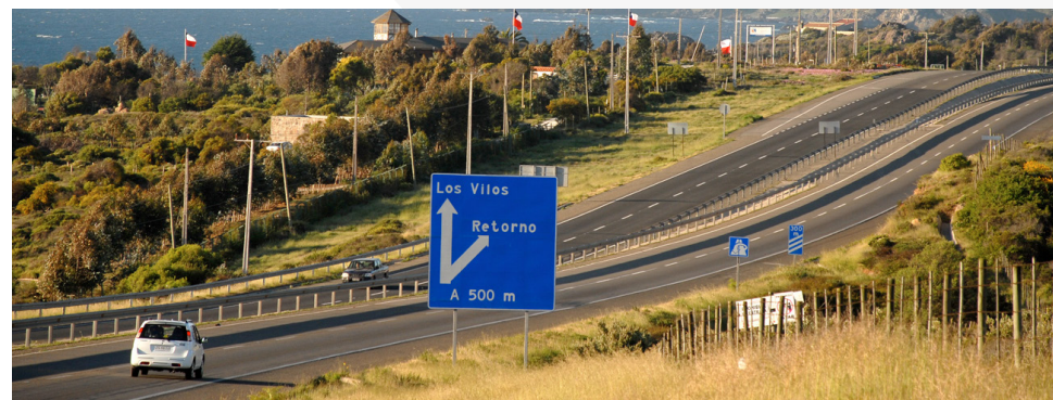
Aconcagua Motorway (Chile).
