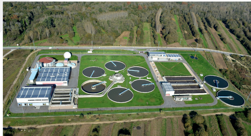
Guillarei Wastewater Treatment Plant in Tui (Spain).
