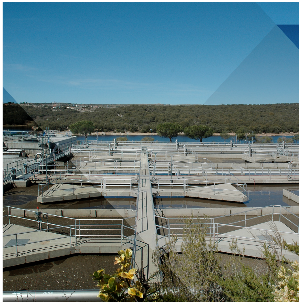
Ávila Wastewater Treatment Plant (Spain).
