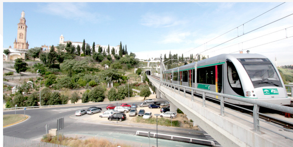
Seville Metro (Spain).
