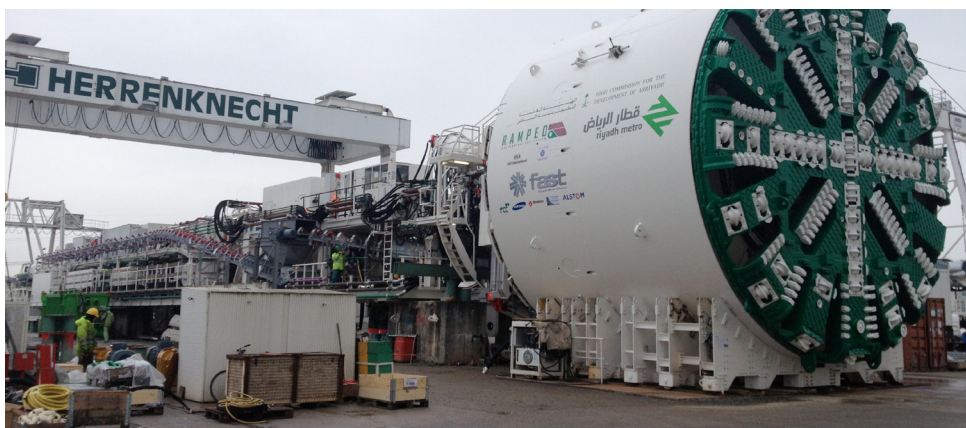
Tunnel boring of Riyadh Metro (Saudi Arabia).
