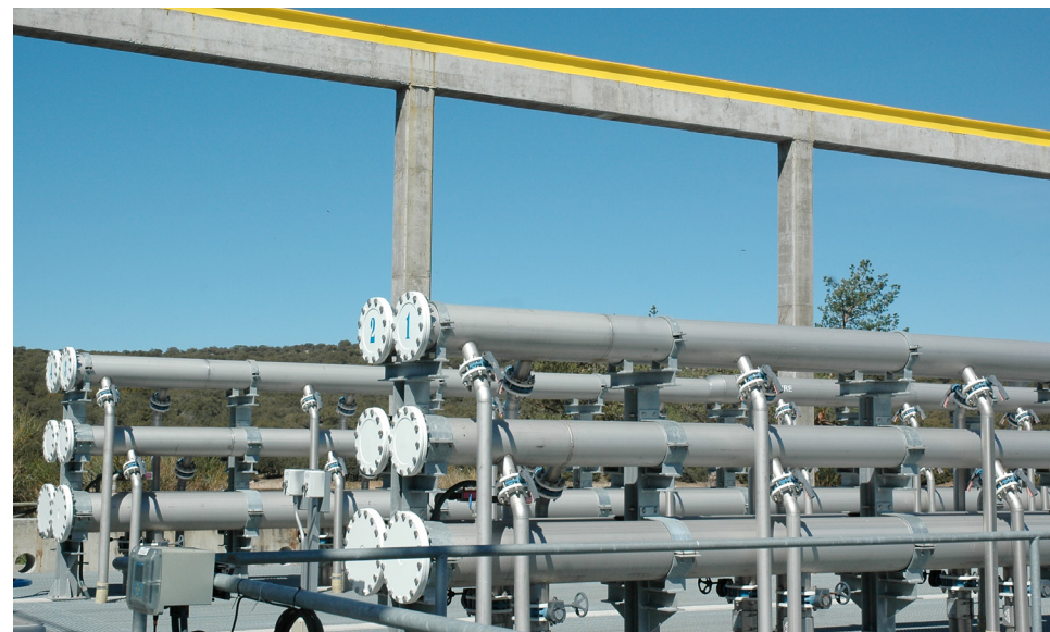
Ultrafiltration membrane bioreactor (MBR).
