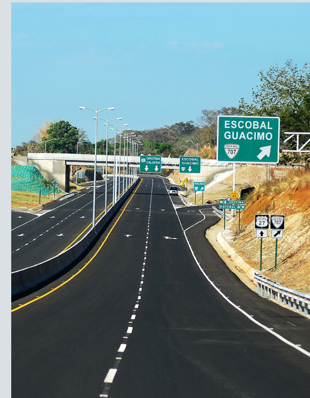
San José Caldera Motorway, Costa Rica
