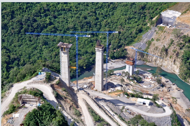
Piers for San Marco Viaduct, Mexico
