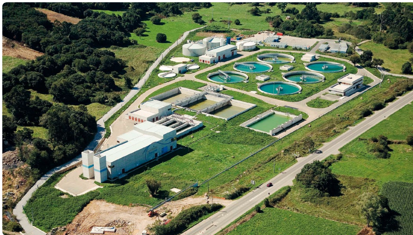
WASTEWATER TREATMENT PLANT, SAN PANTALEÓN, SANTANDER.
