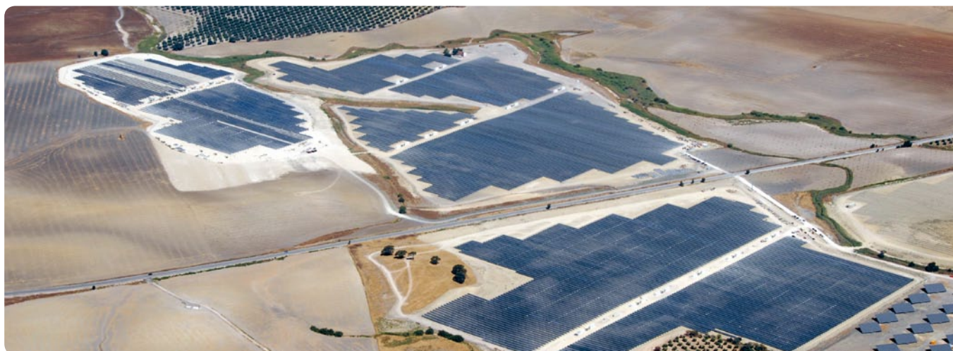
PHOTOVOLTAIC SOLAR FARM, ESPEJO, CÓRDOBA.
