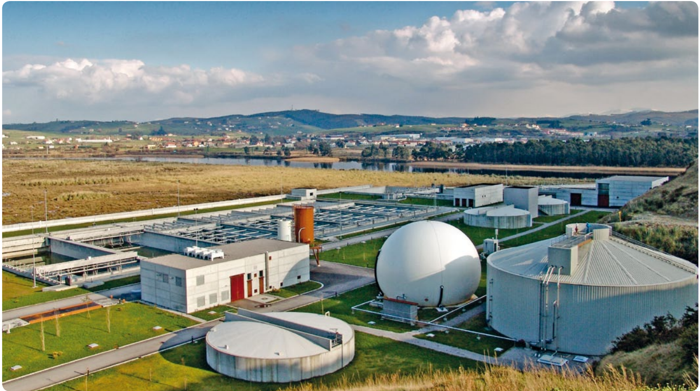
WASTEWATER TREATMENT PLANT, SUANCES, CANTABRIA.
