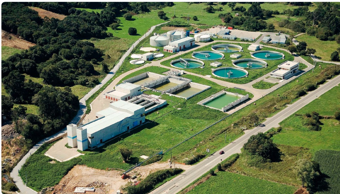
WASTEWATER TREATMENT PLANT, SAN PANTALEÓN, SANTANDER.
