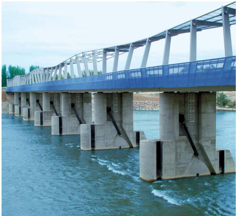
■ **Section VI of the water supply system from the Cenajo reservoir to the Taibilla Canal Association** (Murcia). A section of the trunk system between the Altiplano bypass and the connection to the Campotejar water treatment plant. It is 34.7 metres long and includes three energy recovery installations.
