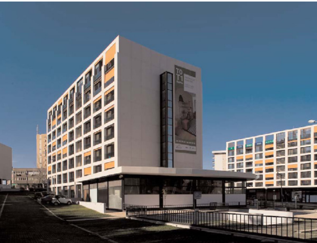
Housing at Cruz de Celas, Coimbra. Portugal
