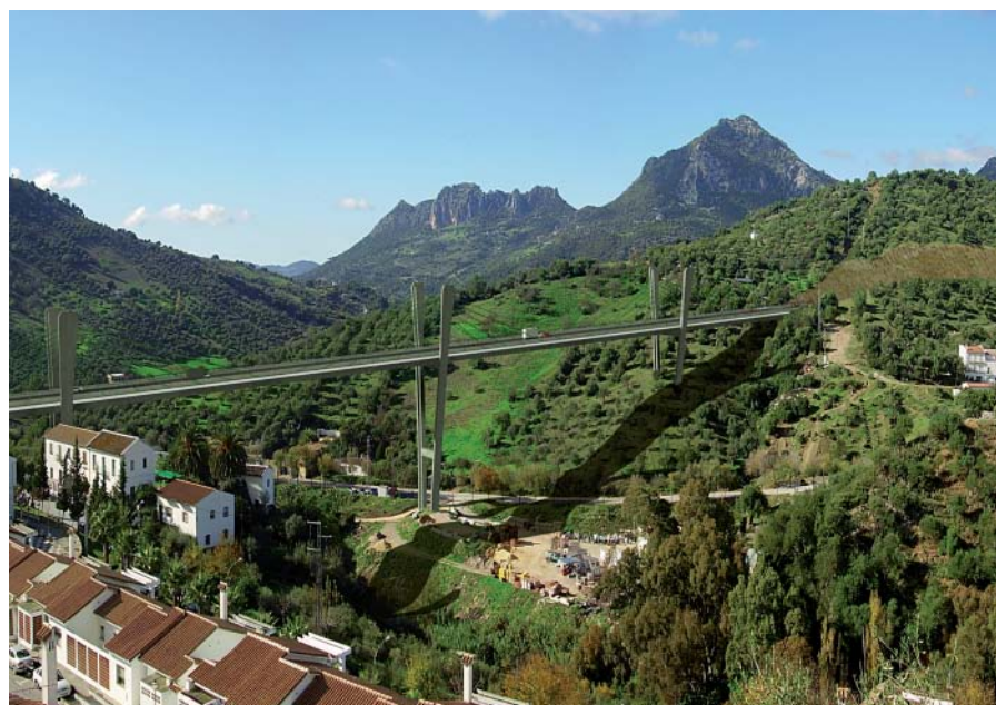
West relief road viaduct in Ubrique. Cádiz
