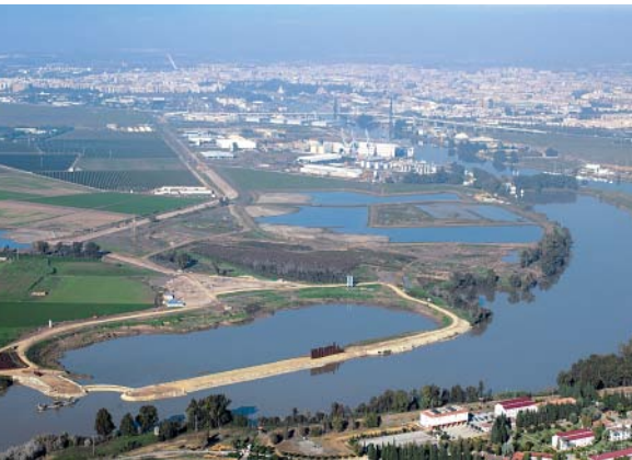
Seville Harbour lock
