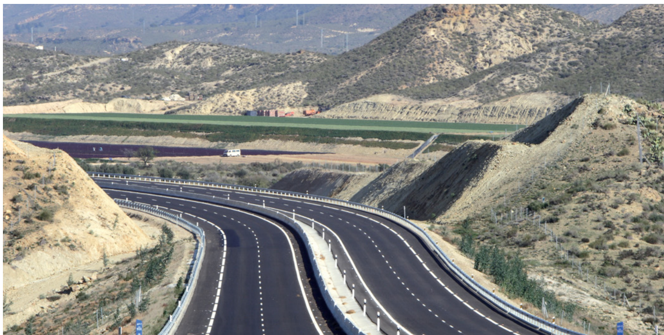
Canero Viaduct. Cantábrico motorway. Querusas - Otur section
