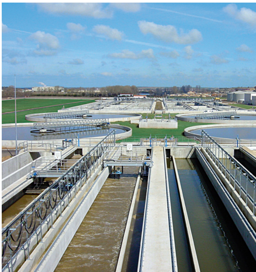
Wastewater treatment plant. Salamanca
