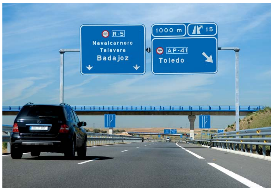
Radial 5 dual carriageways. Madrid
