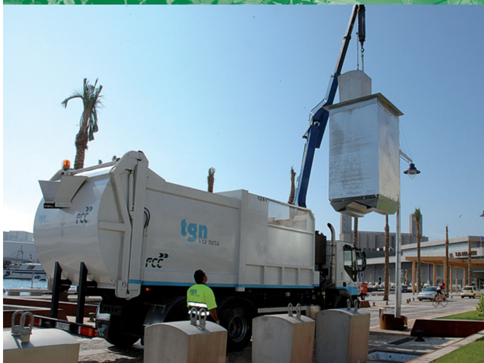
Solid urban waste pick-up from containers installed below street level. Tarragona
