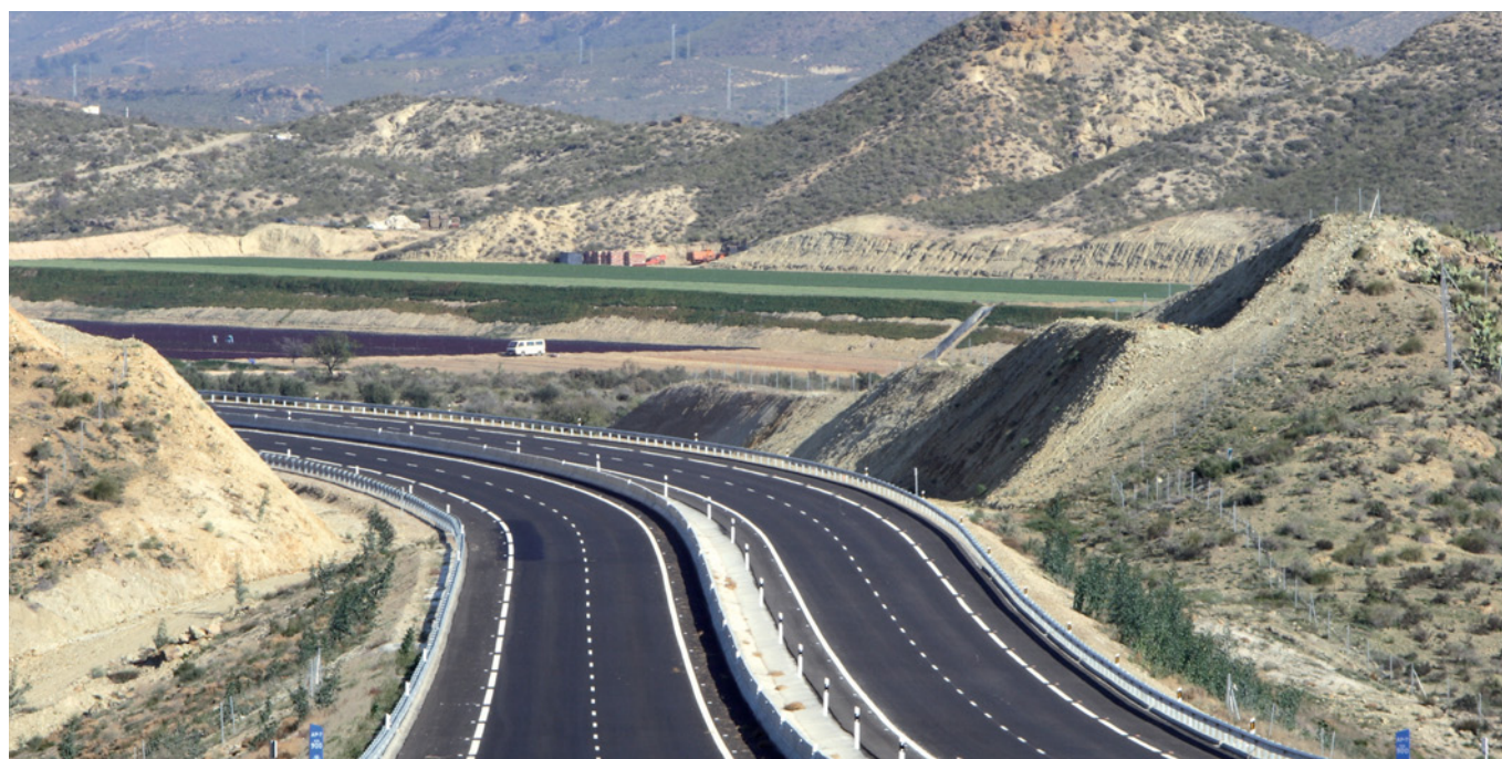
Canero Viaduct. Cantábrico motorway, Querusas - Otur section
