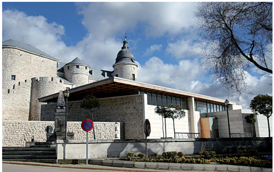
Refurbishment of the Archives of Simancas, Salamanca
