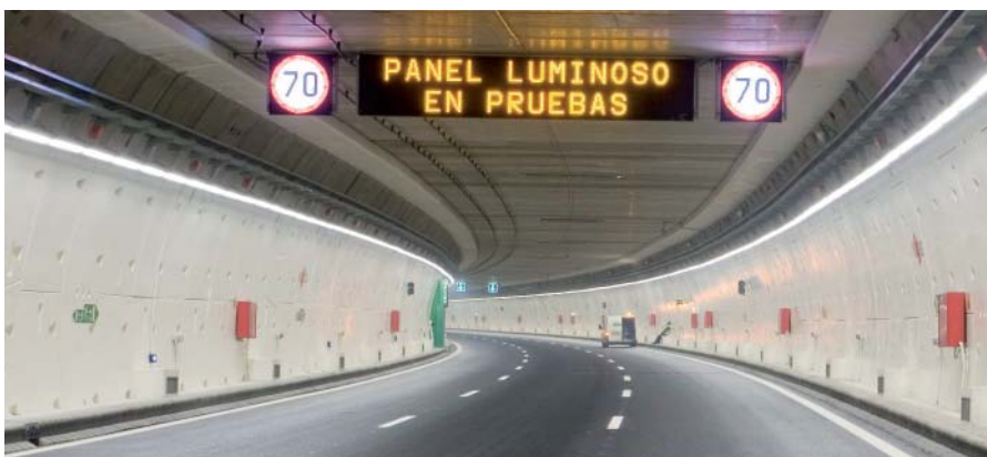
M-30 south bypass tunnel. Madrid
