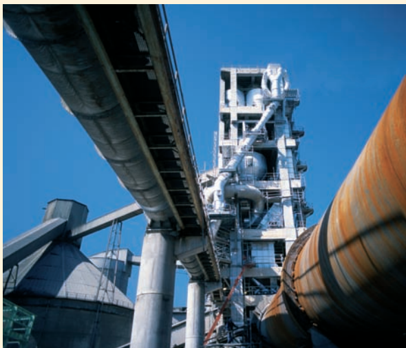
Cementos Lemona factory. Vizcaya
