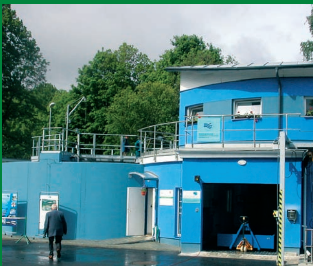
SmVak. Water management. Czech Republic
