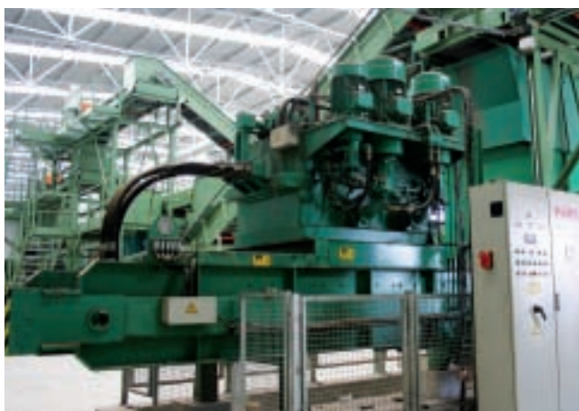
Solid urban waste treatment plant. Tudela. Navarra
