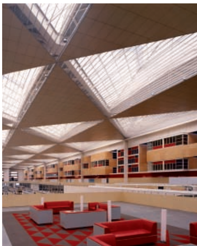
Delicias intermodal transfer facility. Zaragoza
