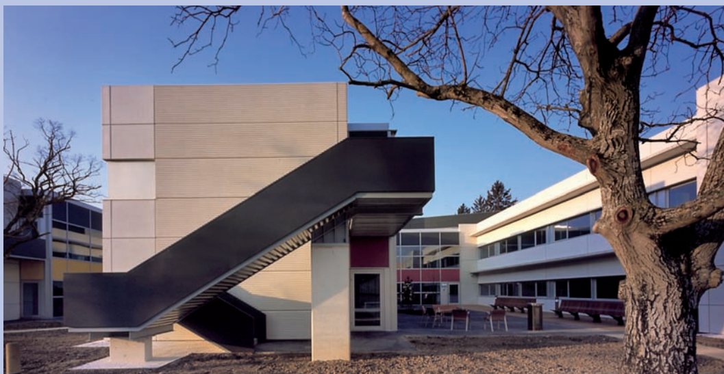
Centre for the mentally handicapped, Pamplona, Navarra
