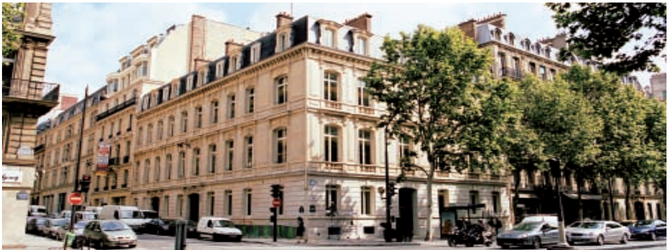
Building at boulevard Haussmann. Paris
