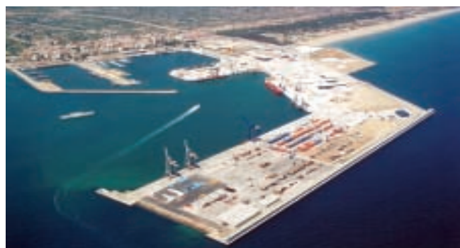
Multipurpose terminal in Castellón
