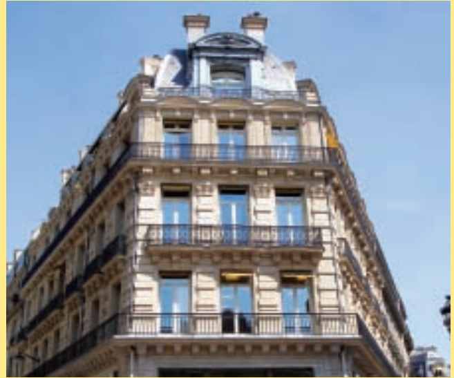
Property. Building at rue Pyramides. Paris
