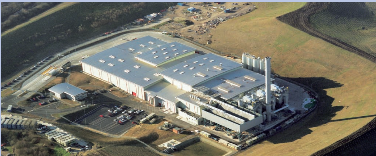
Thermal waste treatment plant. Alington, United Kingdom.
