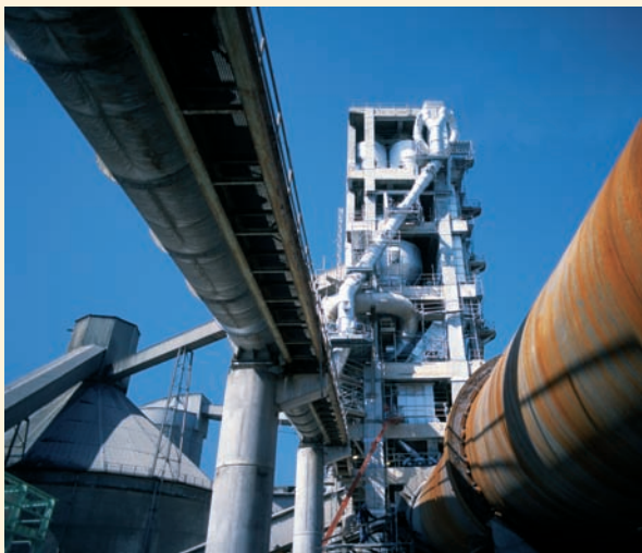
Cementos Lemona factory. Vizcaya
