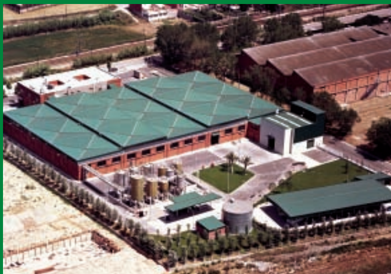
Transfer plant in Montmeló. Barcelona
