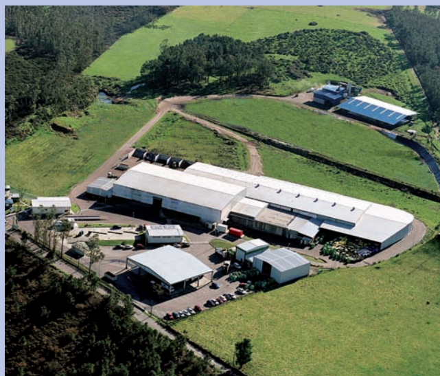
Solid urban waste treatment plant. Barbanza
