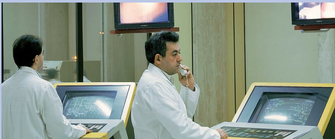
Cement factory control room in Olazagutia, Navarra
