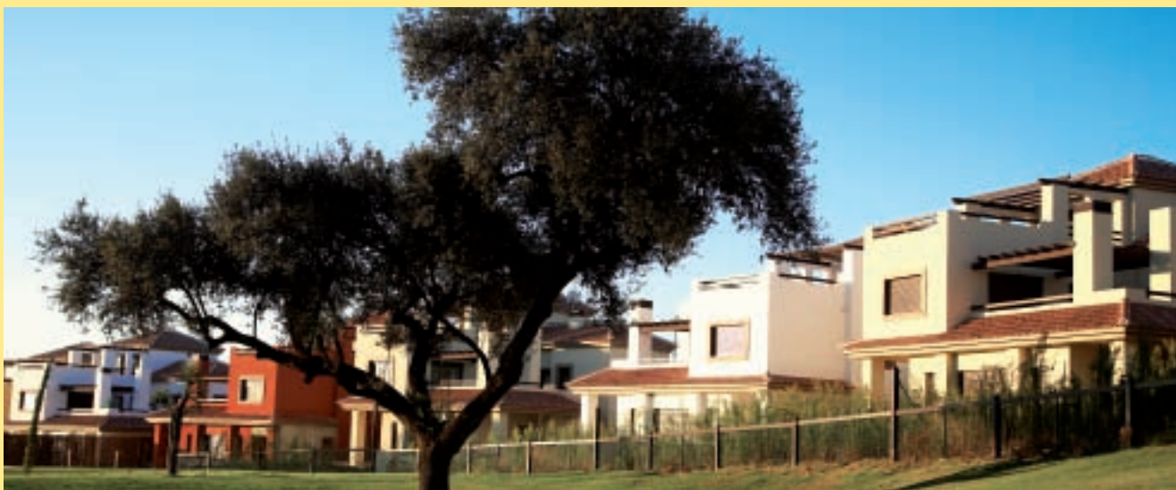
Housing development. Guillena. Sevilla
