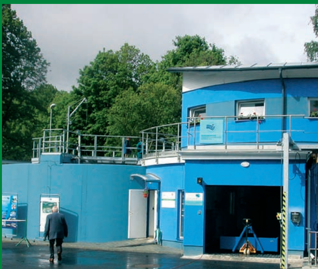
SmVak. Water management. Czech Republic
