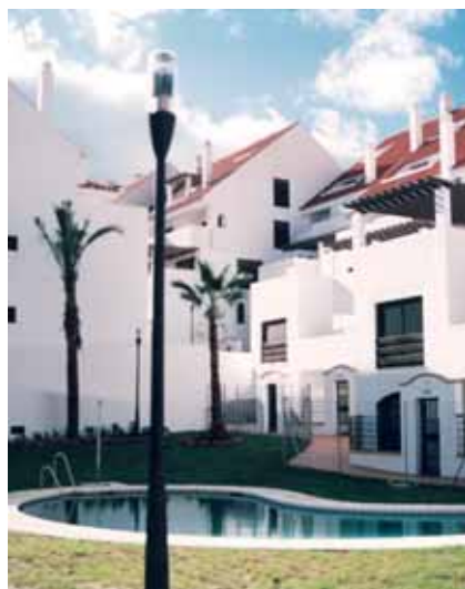
La Maestranza housing complex in Marbella. Málaga
