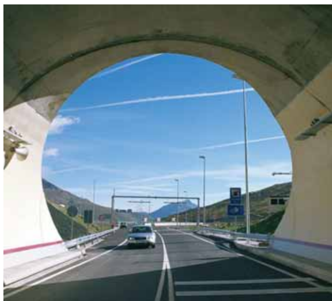
Sóller tunnel concession. Palma de Mallorca
