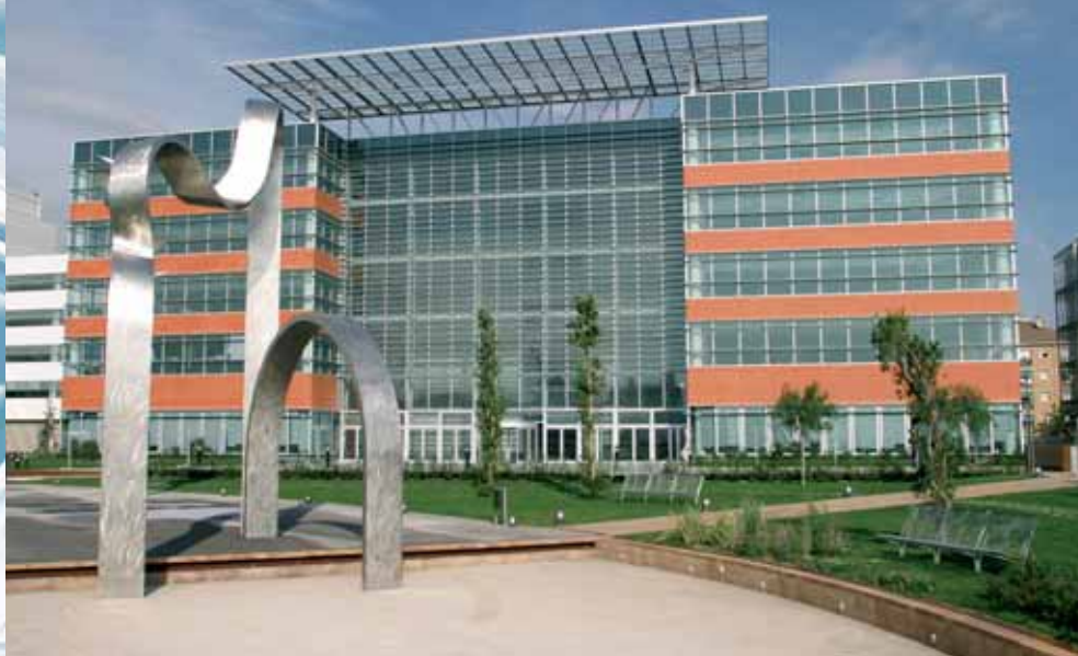
World Trade Center offices in Cornellà. Barcelona
