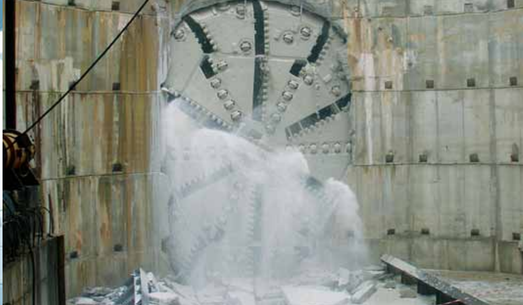
TBM on Line 9 of the Barcelona underground
