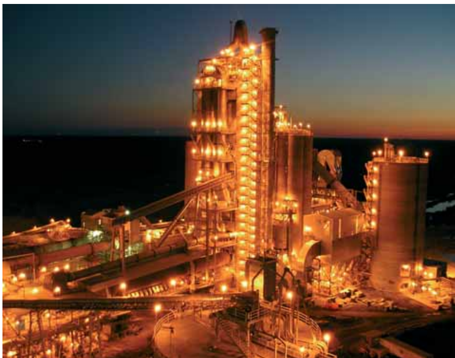
Harleyville cement factory. South Carolina. USA
