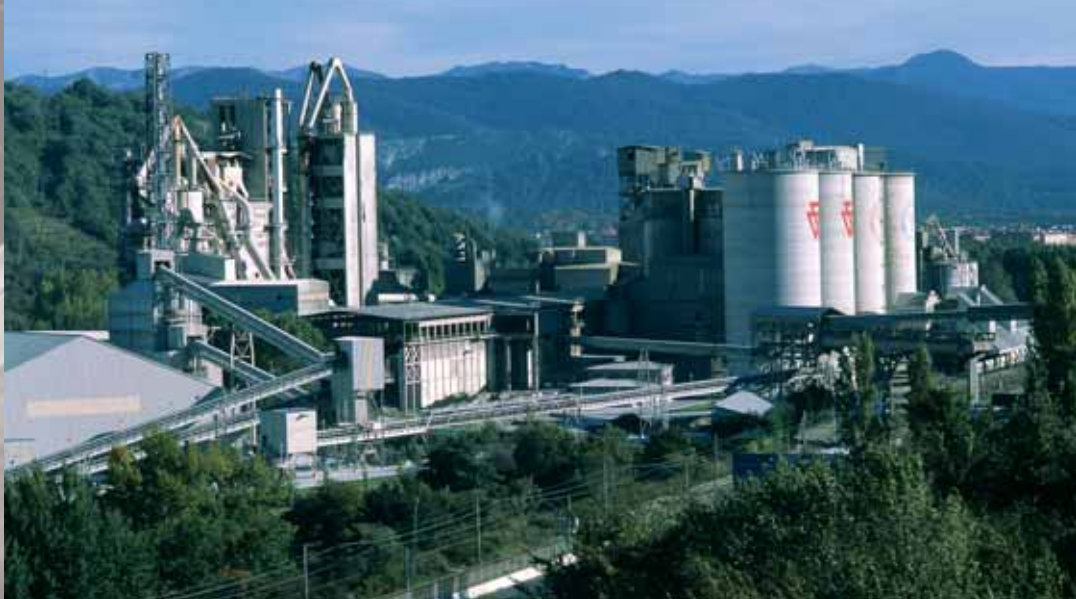
Olazagutía cement factory. Navarra
