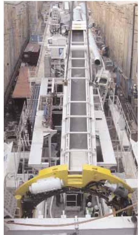
In late December the boring work for the Guadarrama tunnels was completed. These tunnels are part of the Soto del Real-Segovia section of the high speed train line. The work consisted of a 28.4 km stretch with an interior diameter of 8.5 m.
