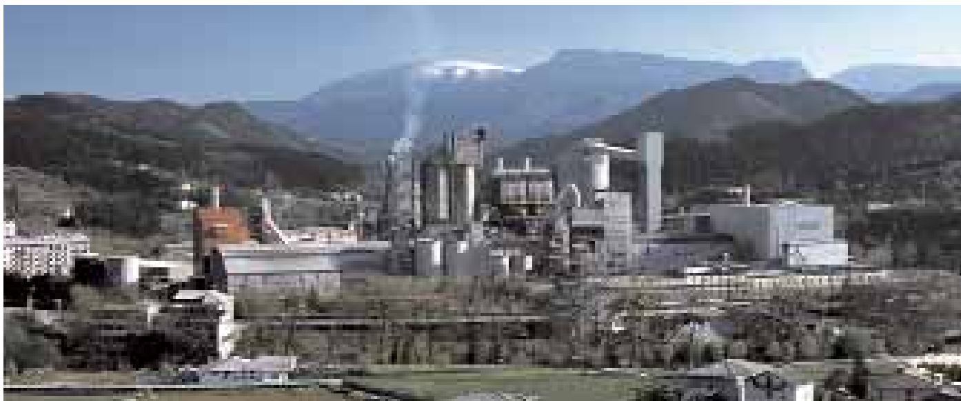
■ Cement factory in Lemona. Vizcaya
