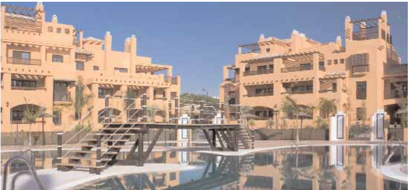
■ Residential complex in Marbella-Estepona. Málaga
