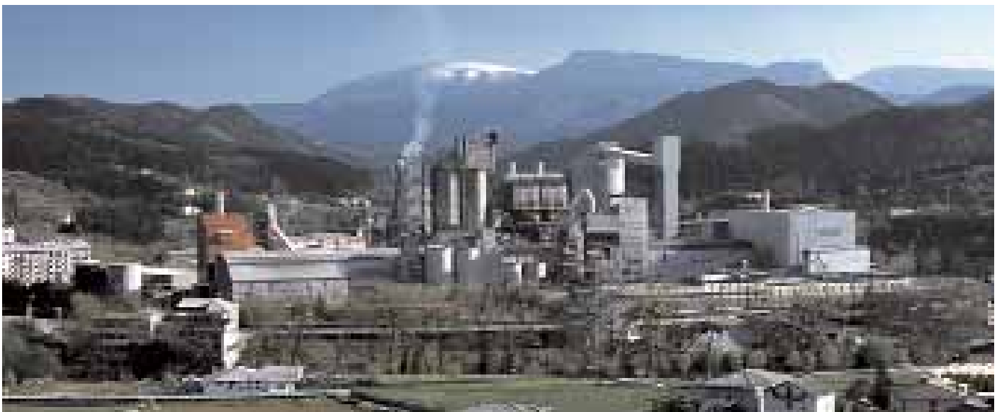
Cement factory in Lemona. Vizcaya
