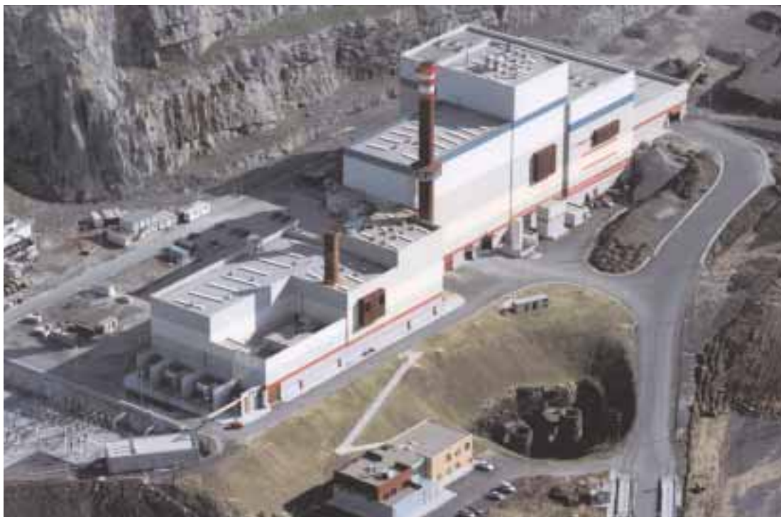
■ Solid waste treatment plant in Zabalgarbi, Vizcaya
