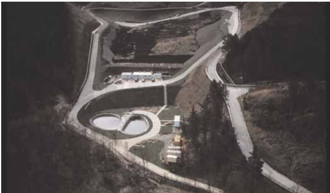
■ Industrial waste treatment plant in Constati. Tarragona
