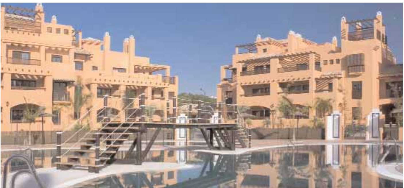
■ Residential complex in Marbella-Estepona. Málaga
