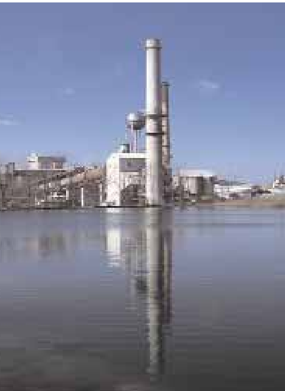
■ Cement factory in Keystone. USA
