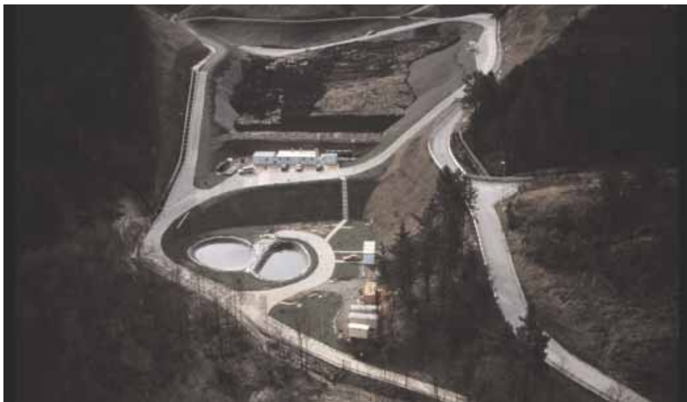
■ Industrial waste treatment plant in Constati. Tarragona
