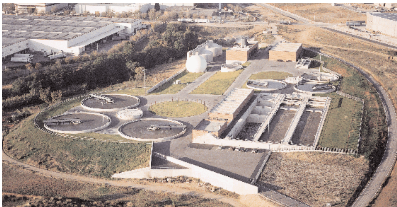
Wastewater purification station. Sabadell. Barcelona
