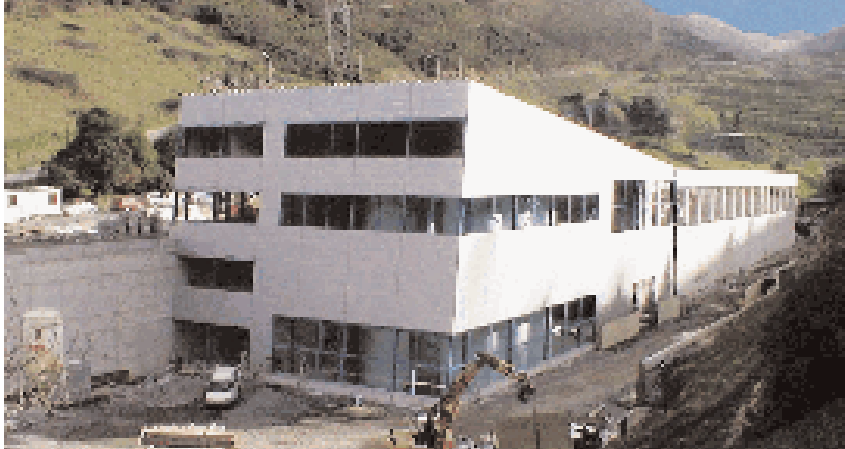
Leachate treatment plant in Artigas. Bilbao.
