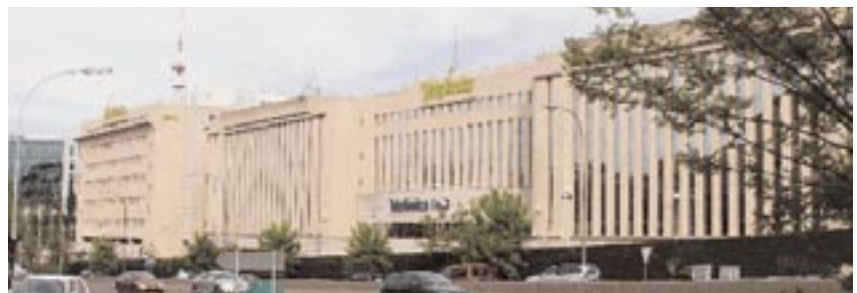
Telefónica's R&D and technology building. Madrid
