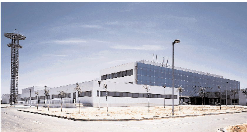
Barcelona Airport. Control centre in Gavá
