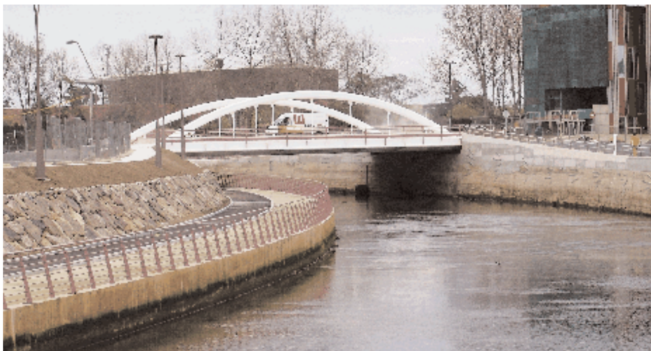
Improvement of the Piles River. Gijón. Asturias
