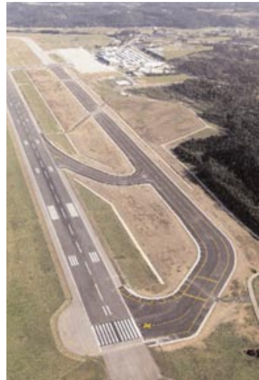
Asturias Airport. Taxiways to pierhead 11
