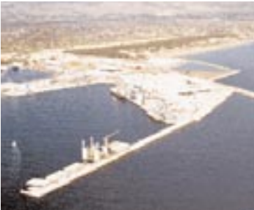
Remodelling the port of Castellón
