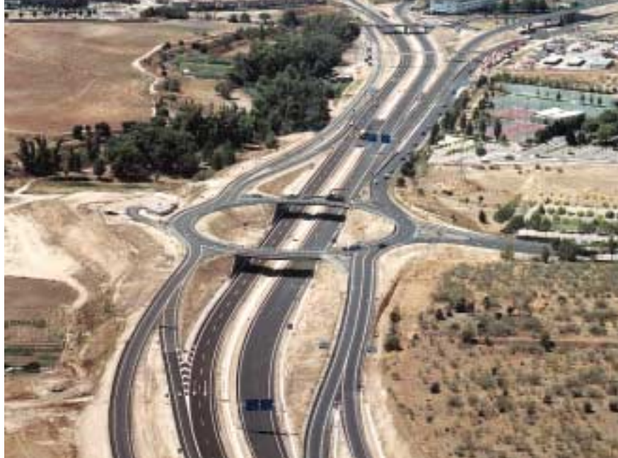
Los Pantanos dual carriageway. Madrid
