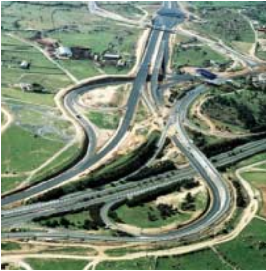
A-6 Freeway, Ávila connection
