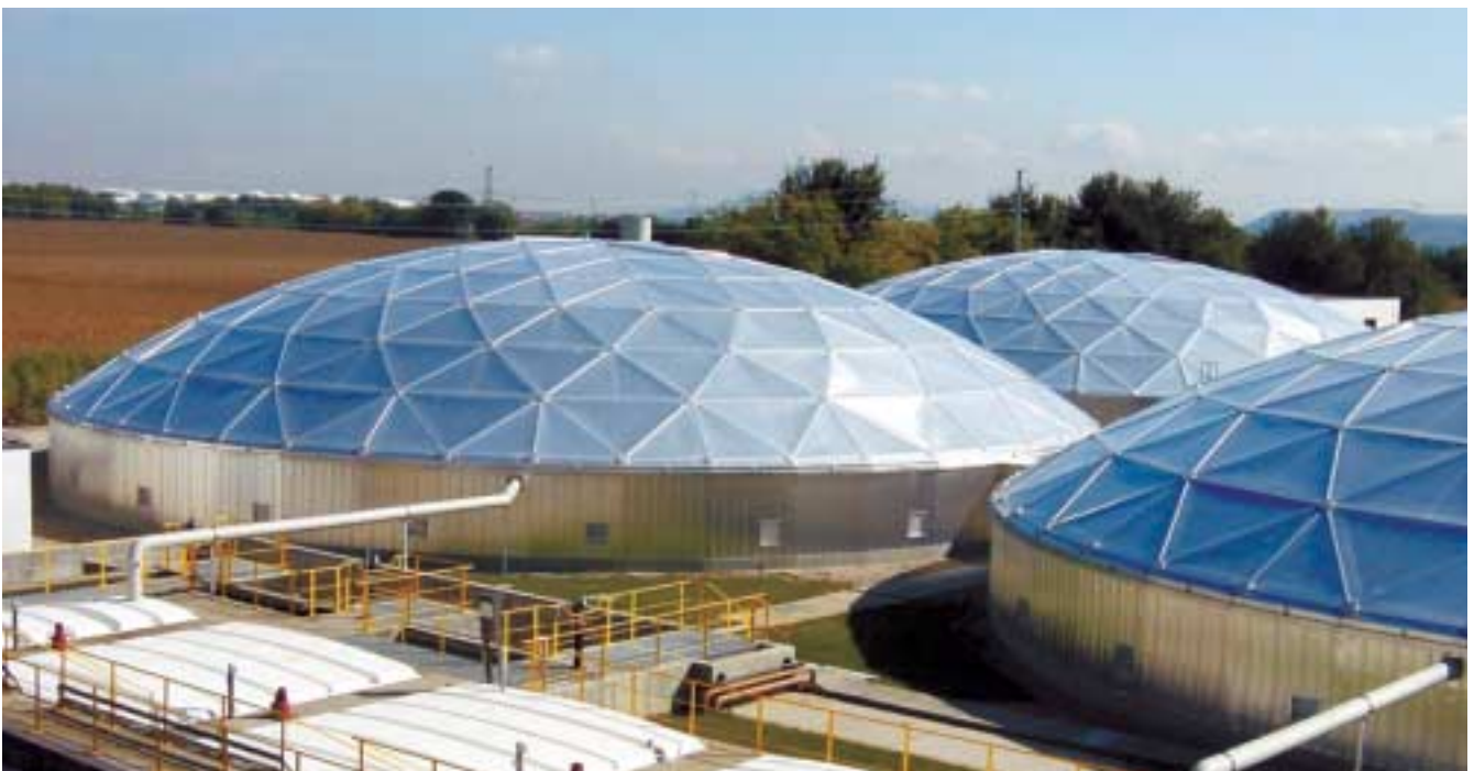
Valmojado wastewater treatment plant in San Fernando de Henares. Madrid
