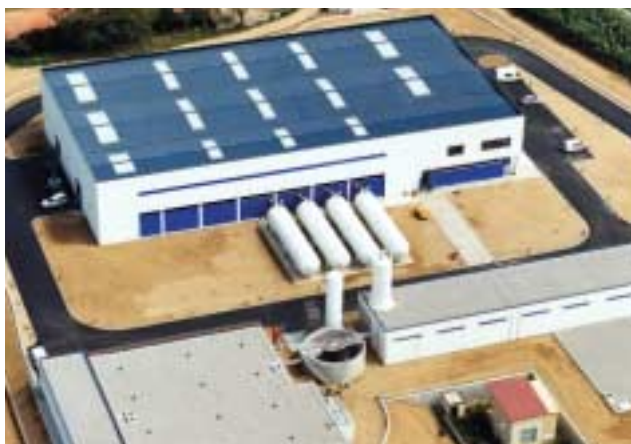
Blanes desalination plant. Girona
