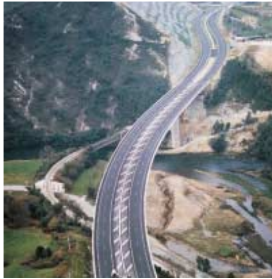
CN-632 Cantábrico Dual Carriageway. Caravia-Llovio section. Asturias
