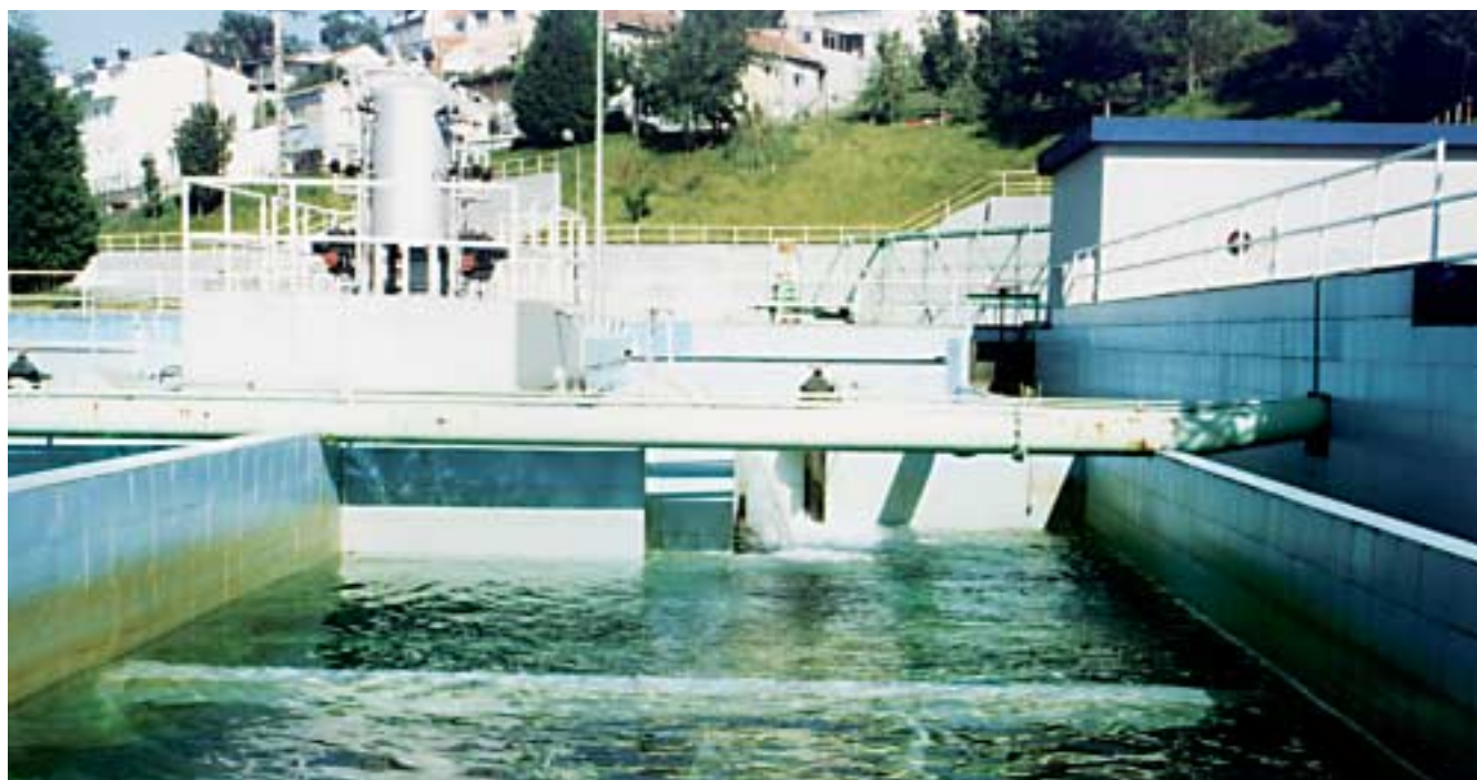
Wastewater treatment plant in, Río Lagares, Vigo. Pontevedra
