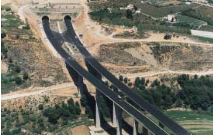
Chillar viaduct and mouth of the Capistrano tunnels. Frigiliana-Nerja section. Málaga
