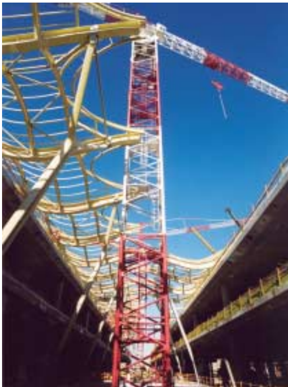
Madrid-Barajas Airport. Structure of new terminal building
