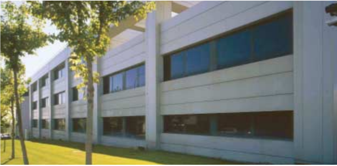
Amper Building. Tres Cantos. Madrid
