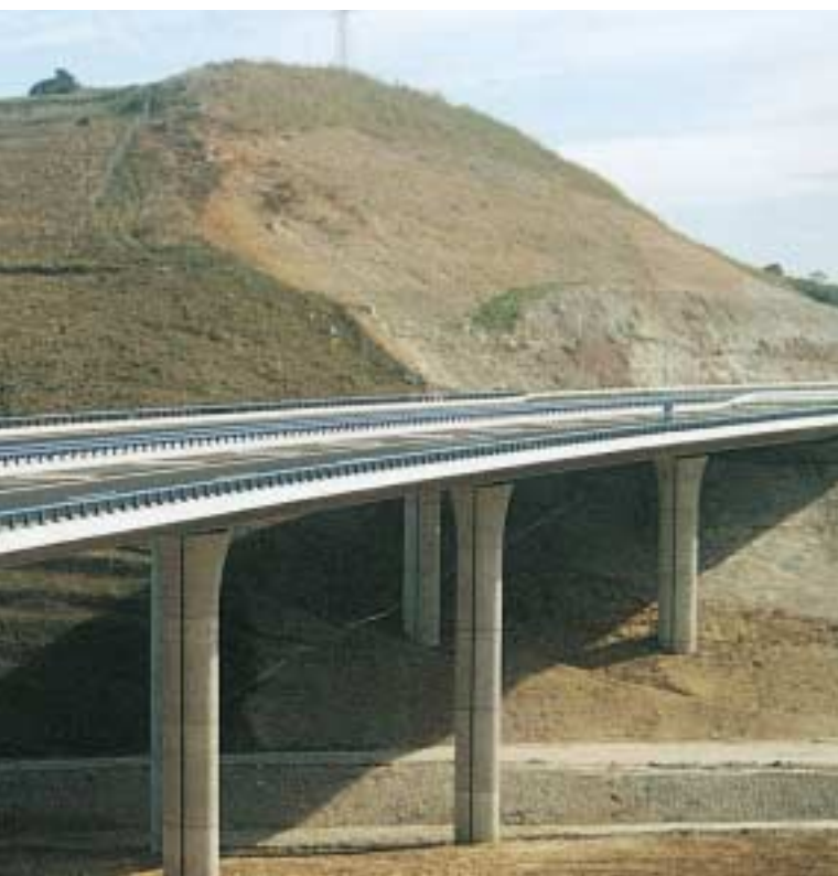
Acebo Viaduct on the Cantábrico Dual Carriageway. Asturias
