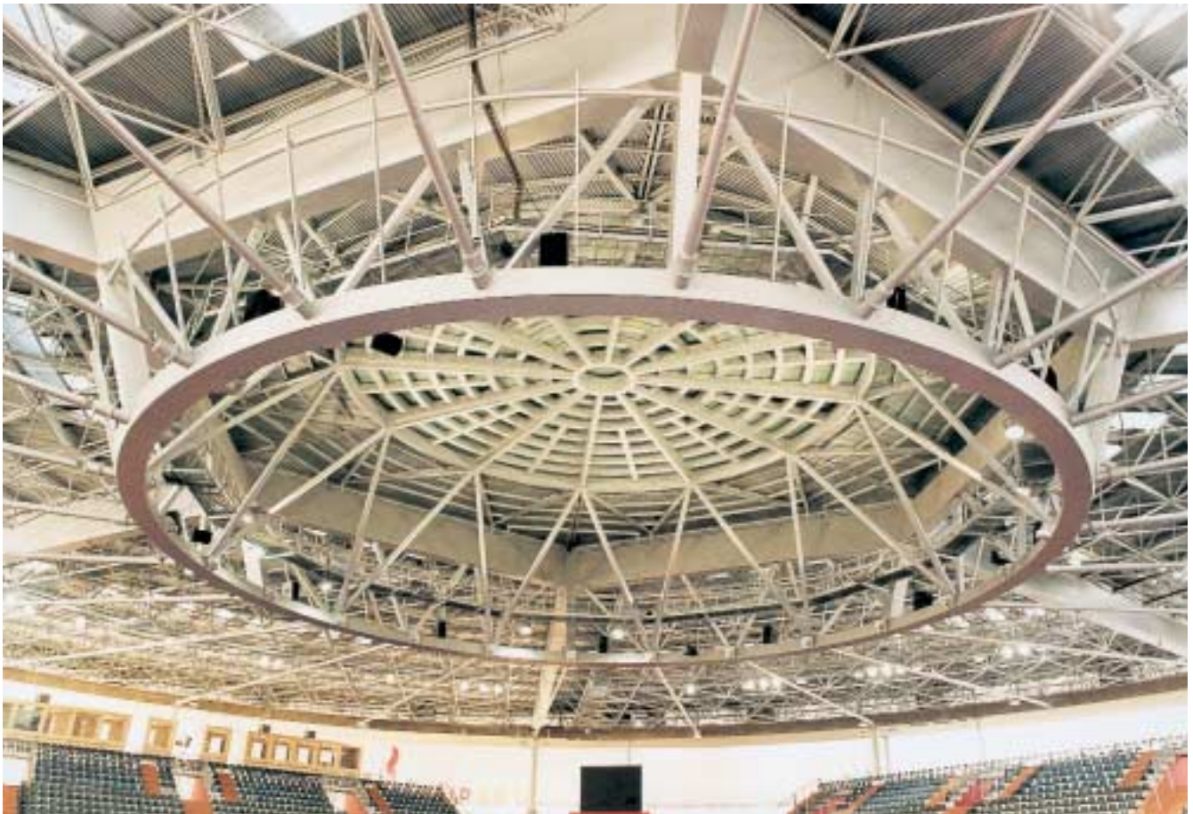
Roof of rockodrome at the Casa de Campo. Madrid
