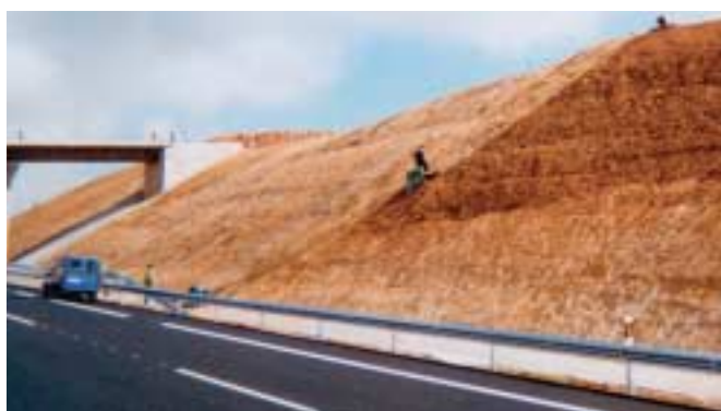
Placement of organic cover on slopes on the Ávila-Villacastín Freeway
