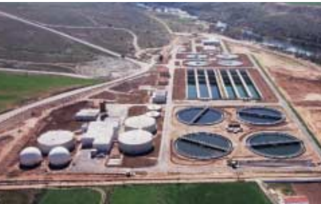
Wastewater treatment plant in Salamanca
