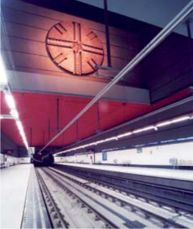
Metrosur. Móstoles exchange. Madrid
