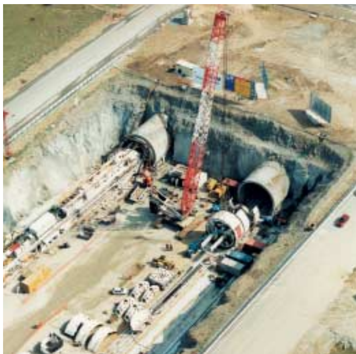
Guadarrama tunnels. High speed train line between Madrid and the north and north-west of Spain
