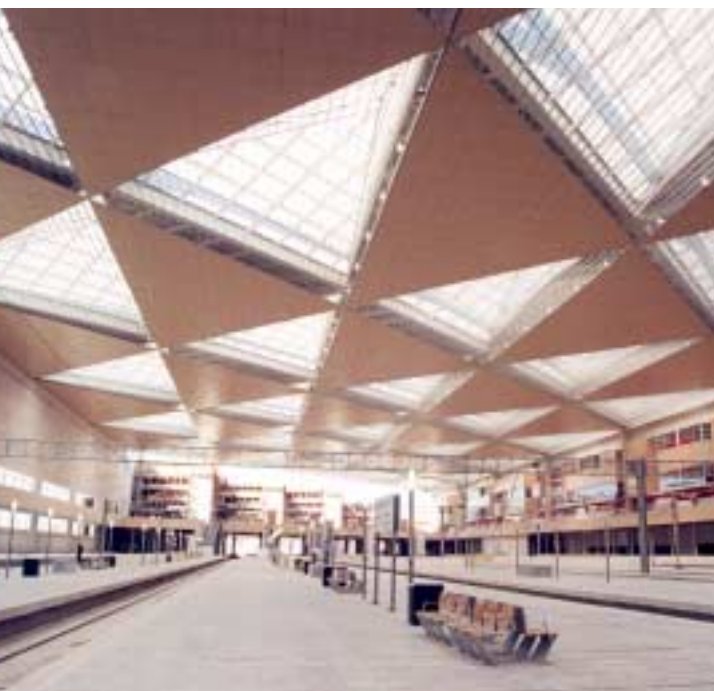
Roof over the Zaragoza-Delicias high speed train station
