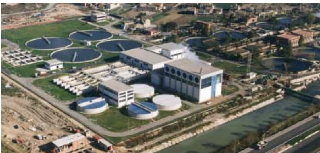
Wastewater treatment plant in Pinedo. Valencia
