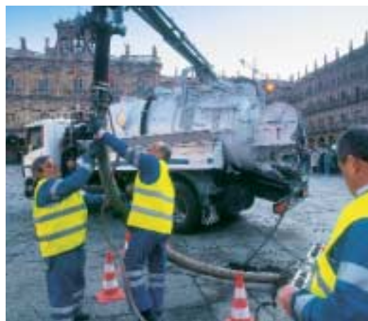
Sewer cleaning service in Salamanca
