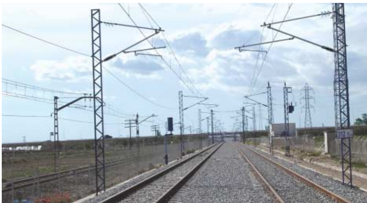
Construction of high speed train line. Zaragoza-Pina de Ebro section
