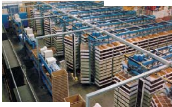
Automatic picking installations.
