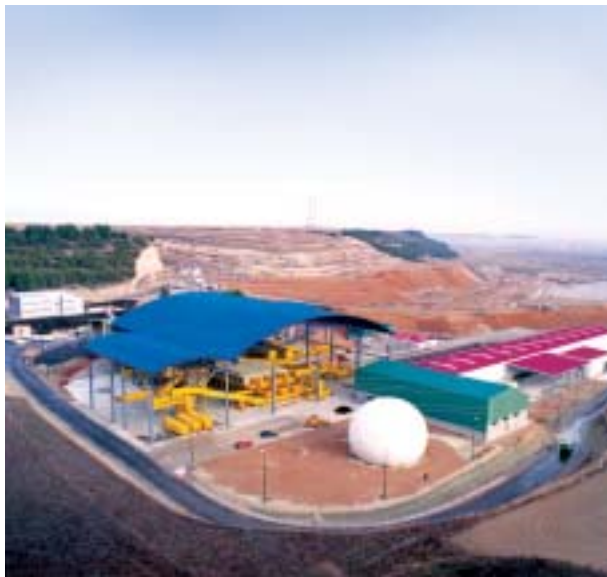
Waste recycling plant. Valladolid.
