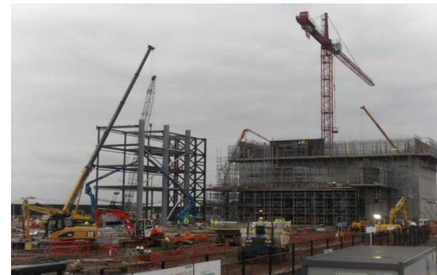
Building in progress (Feb. 2012)
