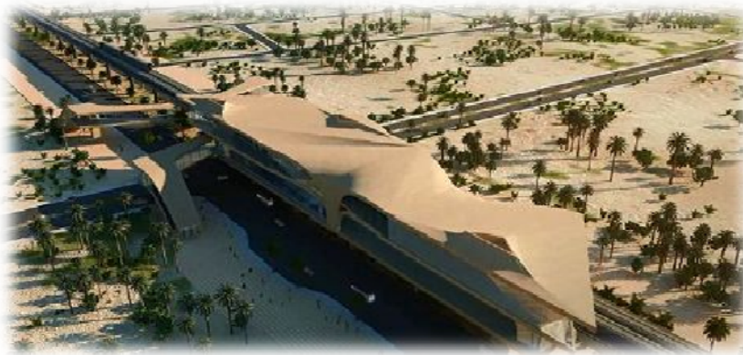
Doha metro (Qatar)
