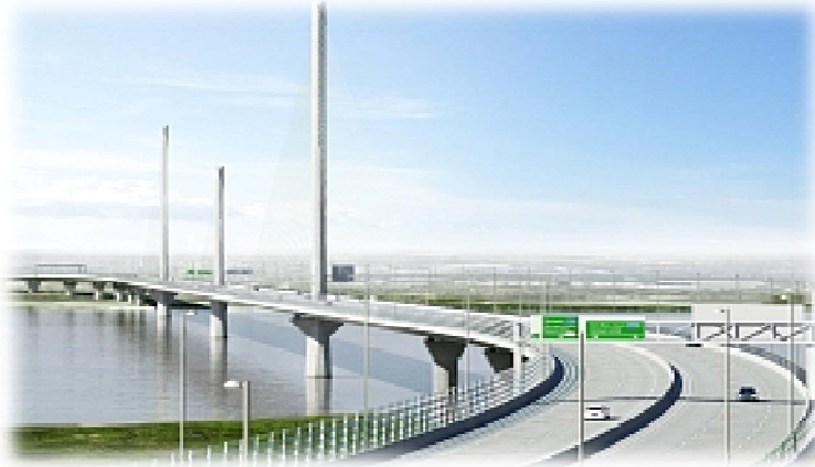
Mersey bridge (Liverpool - UK)
