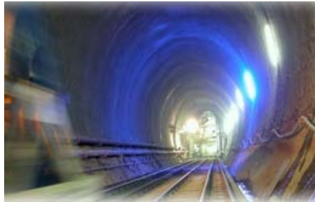
St. Gotthard Tunnel in Switzerland
