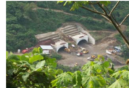
Xicotepec Tunnel in Mexico
