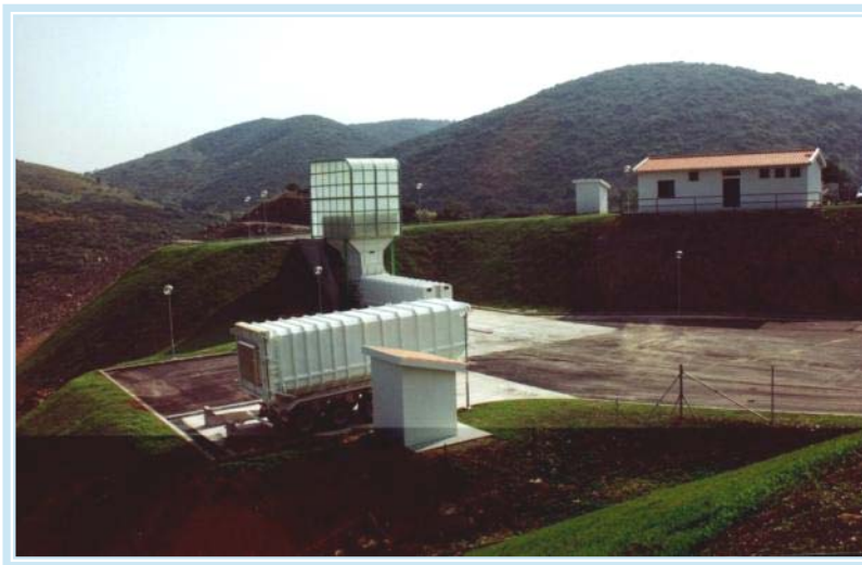
Transfer station in Torre de Moncorvo. Portugal
