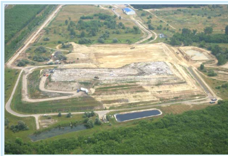
Gyal Controlled Landfill
