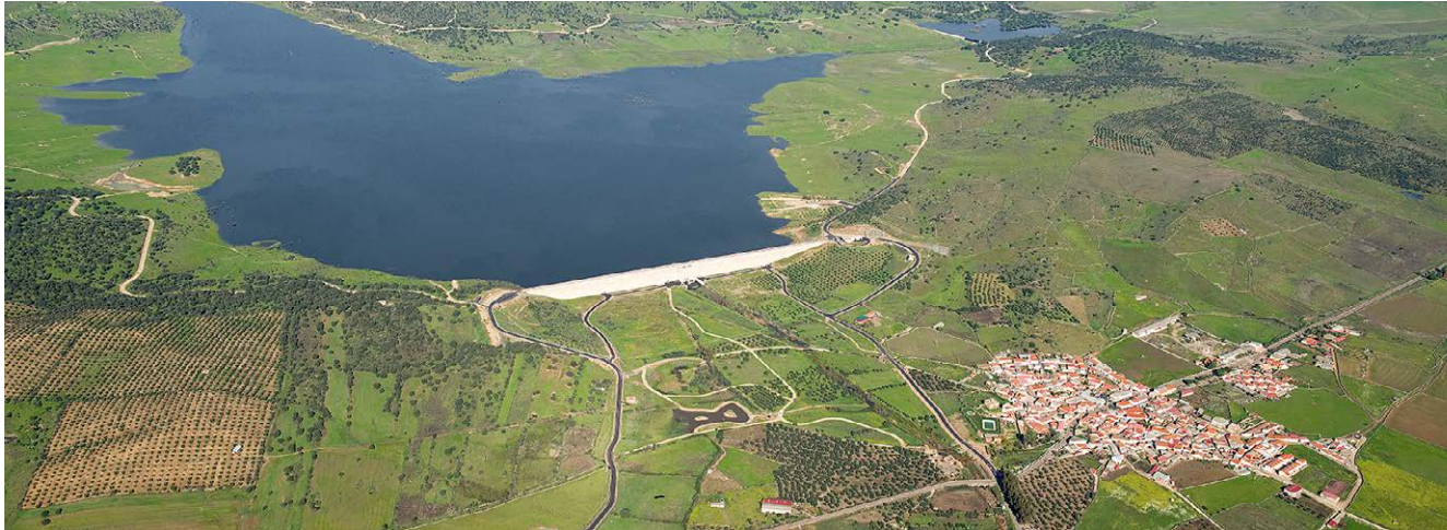
Alcollarín Dam. Cáceres (Spain).
