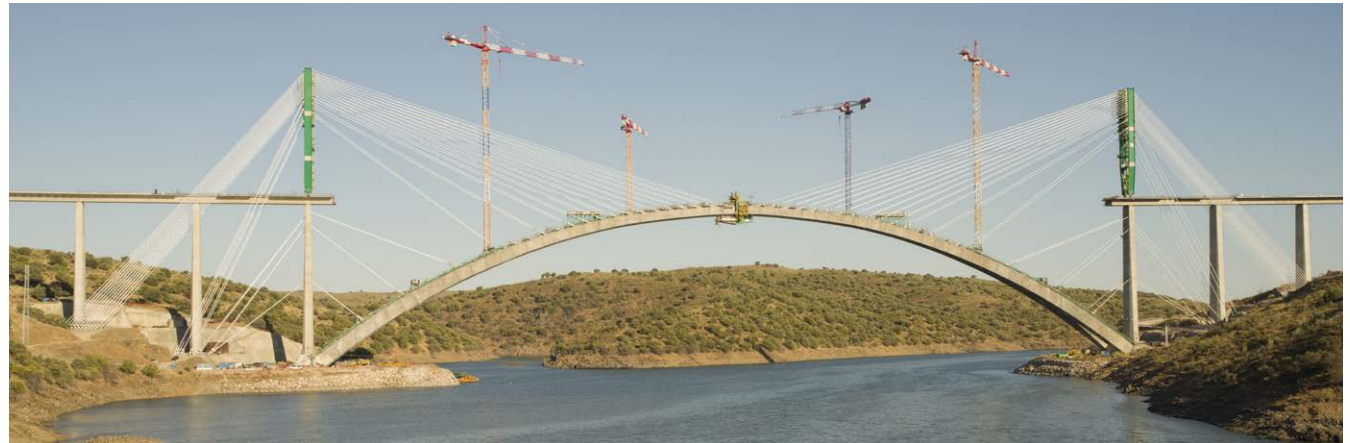
Almonte viaduct (Spain).
