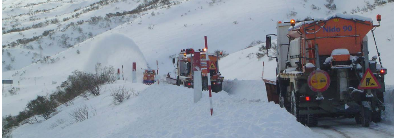
Conservation and maintenance work.
