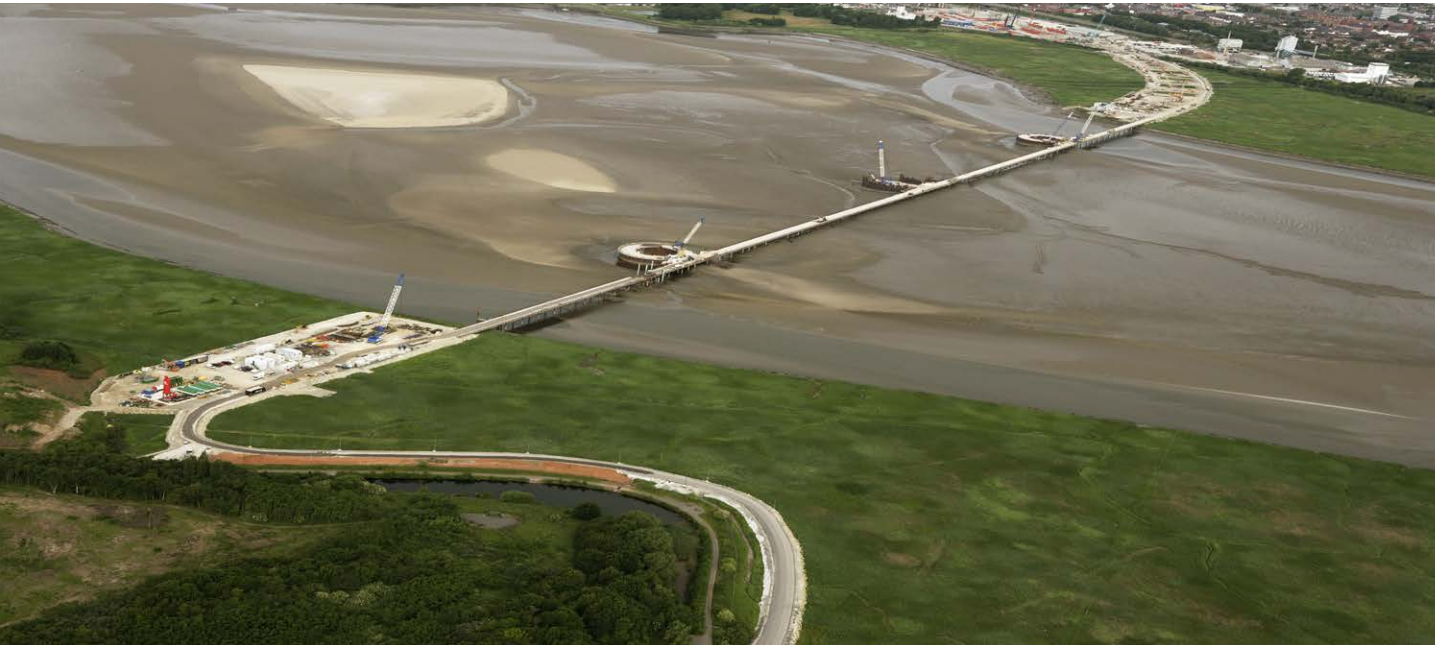
Mersey Viaduct (UK).
