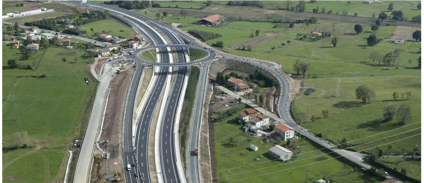
A-8 Dual Carriageway. Solares-La Encina section. Cantabria (Spain).
