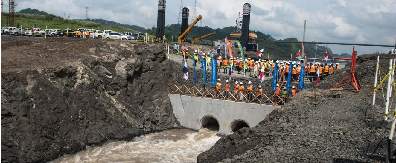
Filling tests of the PAC 4 in the Panama Canal expansion programme (Panama).
