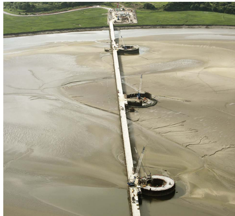
Mersey Bridge (UK).
