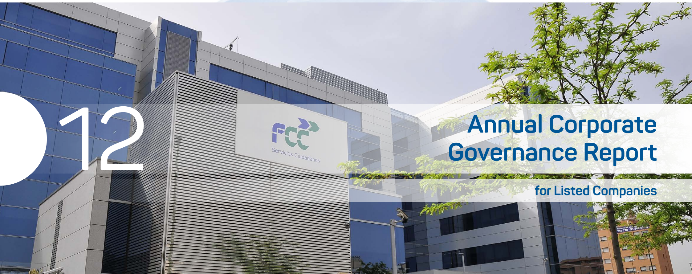
FCC's Main Offices in Madrid (Spain).
