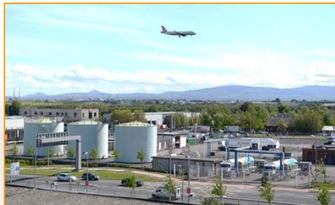
Dublin Airport installations: €33 M
