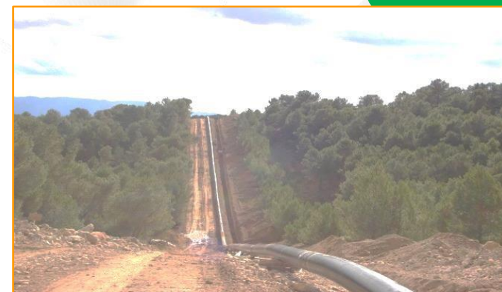
Carso-FCC Gas pipeline Mexico: €225 M
