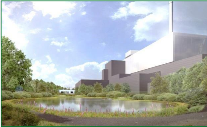
Recycling and energy recovery centre Edinburgh & Midlothian (Scotland)
