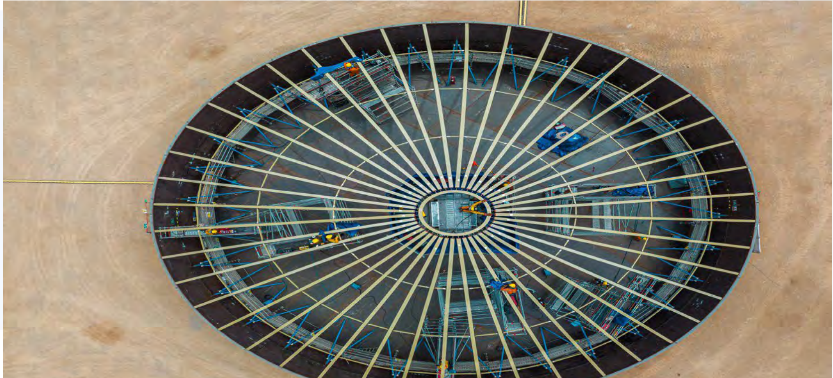
Fuel storage tanks A. International Lima/ Peru
