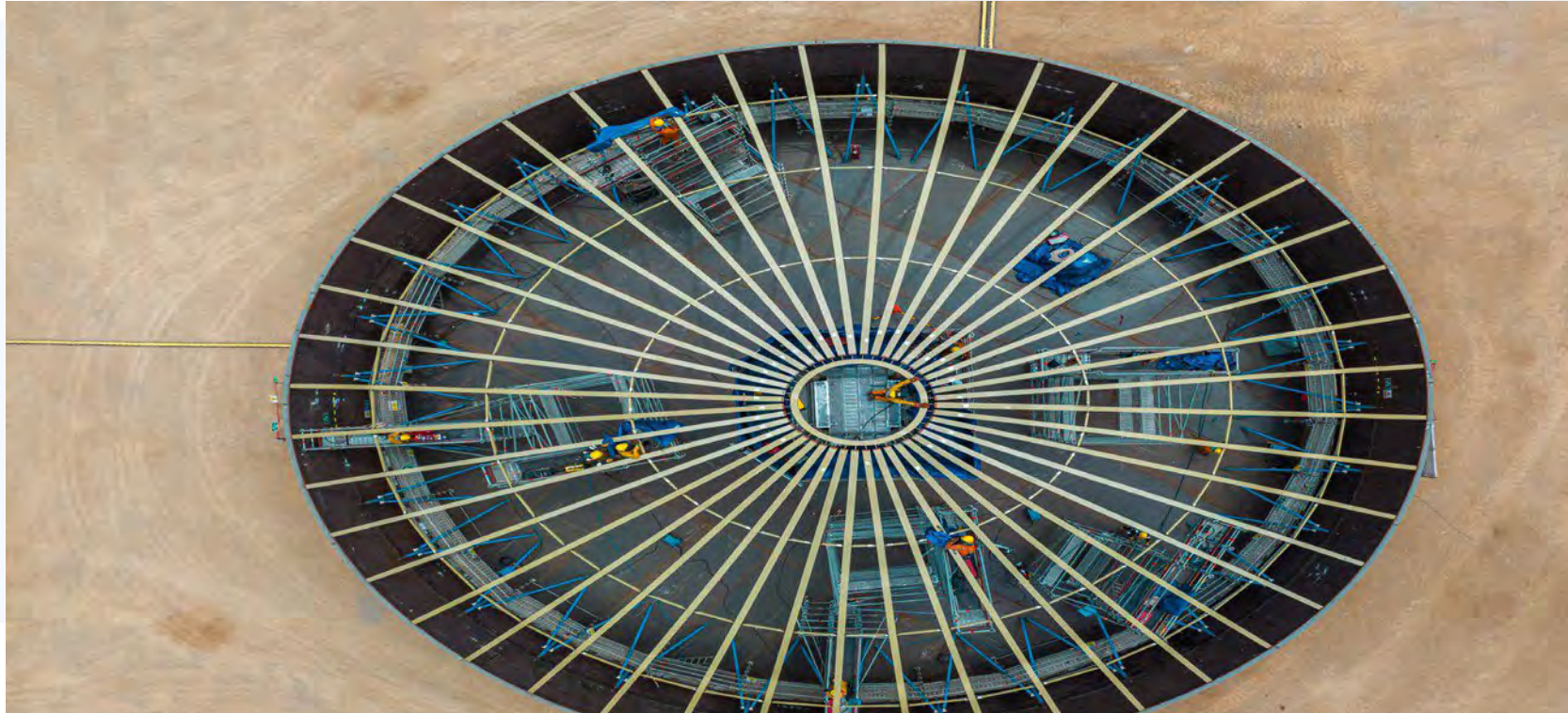
Fuel storage tanks A. International Lima/ Peru
